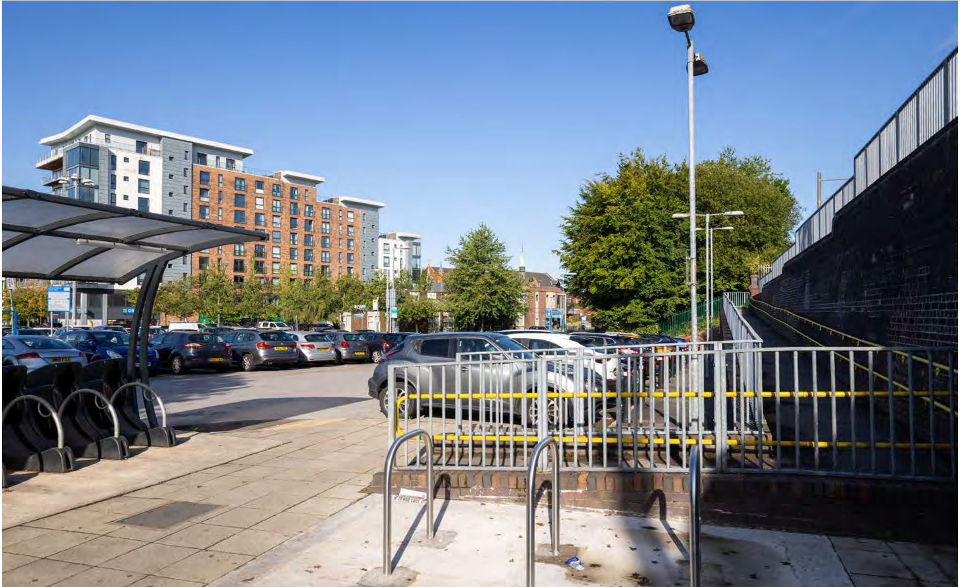
View 1: Baseline photograph | Exit from tram stop on Rectory Lane
