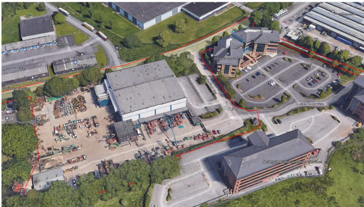
Figure 2: Application site prior to demolition (Google Earth)
