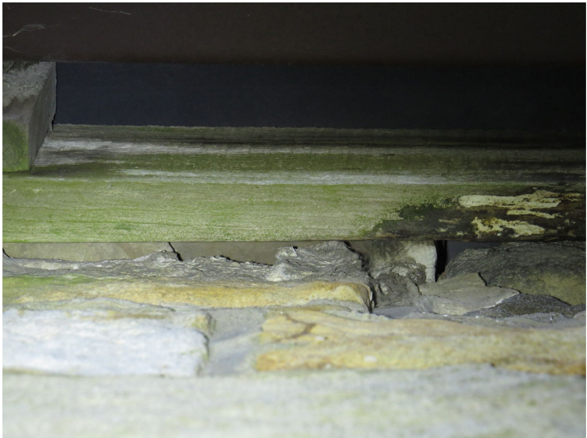
8 - There gaps between timbers and stonework at the eaves.
