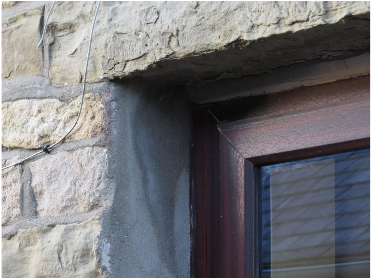
5 - There are no gaps around windows or lintels.
