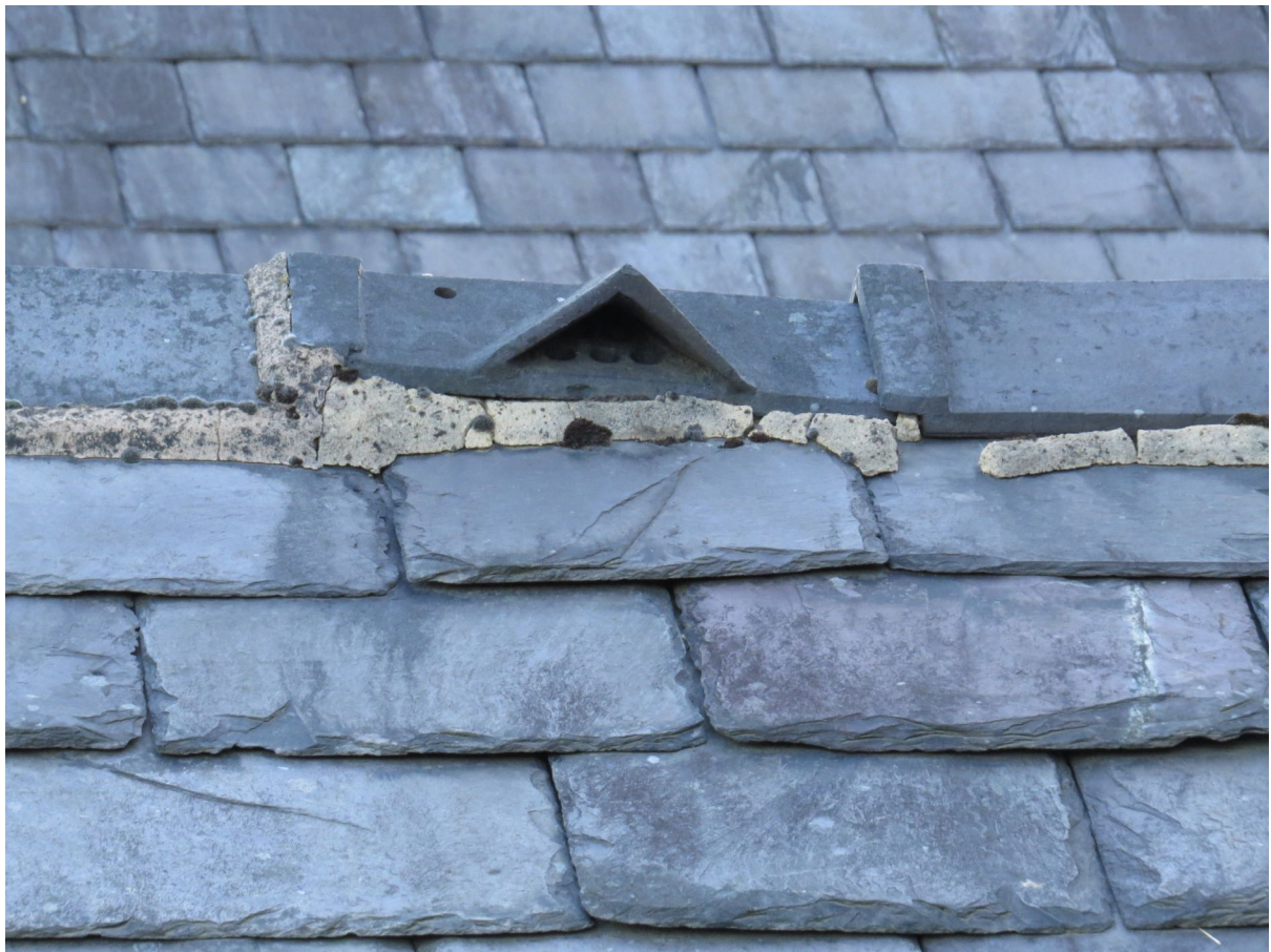
6 - There are gaps beneath roof and ridge tiles on the outbuildings.
