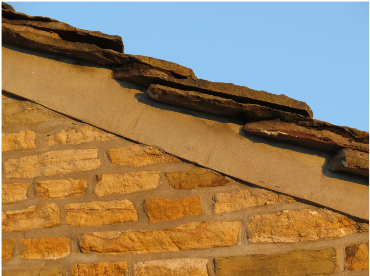
4 - Pointing between stonework and at the verges is in good condition with no gaps.
