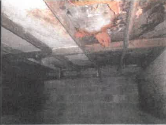
P4 Board lining over stalls
