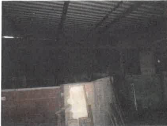
P3 Inside main section, unlined roof
