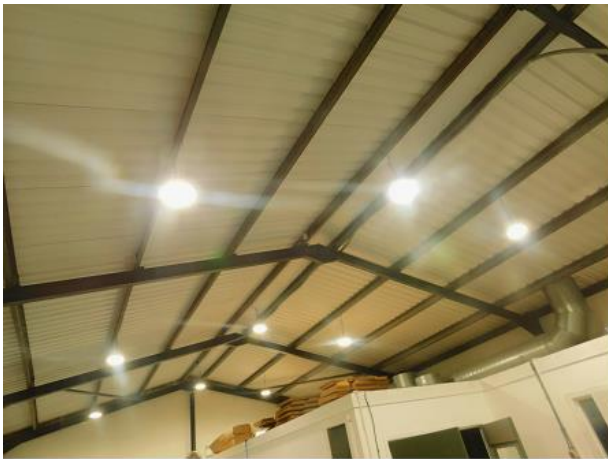
PHOTO 31 Underside of Main Showroom Roof
