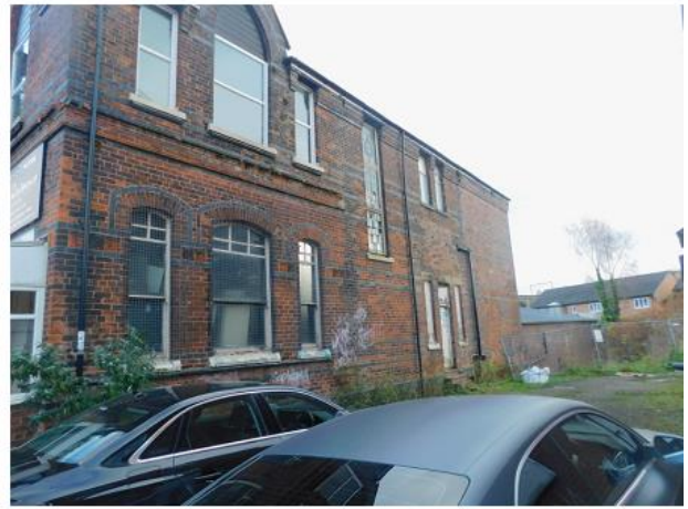
PHOTO 16 View Along Western Elevation
