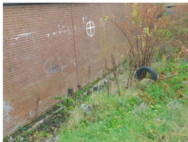
PHOTO 22 Lower Showroom Western Elevation
