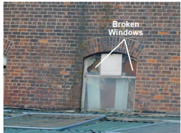
PHOTO 38 Part Southern Elevation of Main Building
