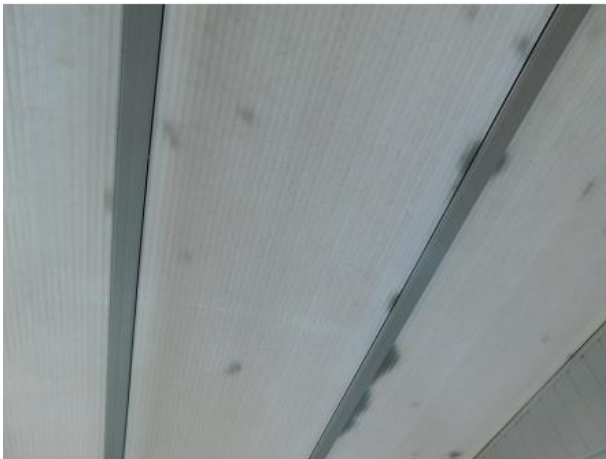
PHOTO 47 Underside of Entrance Roof
