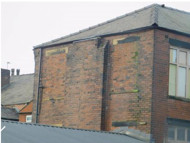
PHOTO 33 South-western Elevation of Main Building
