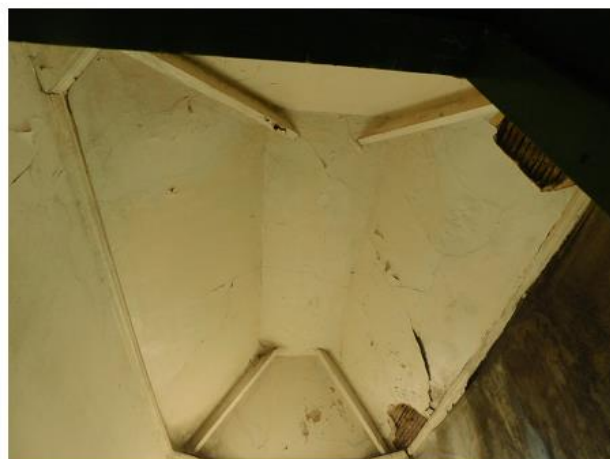
PHOTO 54 Underside of Central Bay Void Roof
