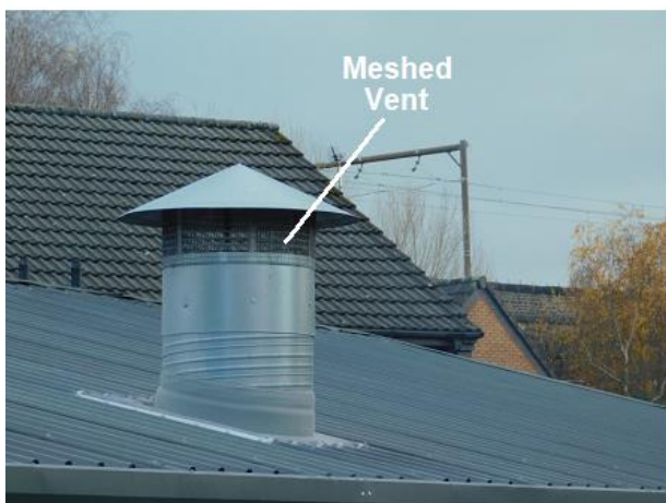
PHOTO 23 View of Vent in Showroom Roof
