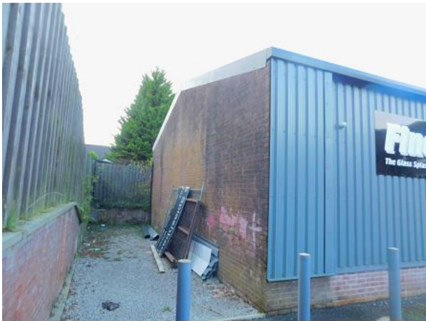
PHOTO 25 Southern Elevation of Showroom
