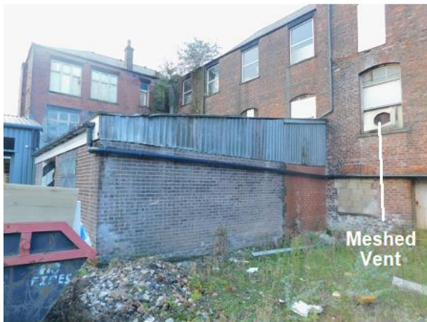
PHOTO 39 Eastern Elevation of Shed
