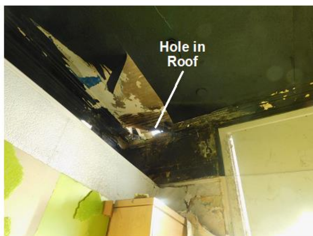
PHOTO 52 Underside of Eastern End of Central Bay Roof
