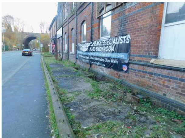
PHOTO 5 View Along Lower Northern Elevation
