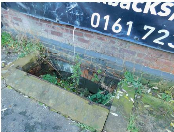
PHOTO 9 North-western Basement Vent
