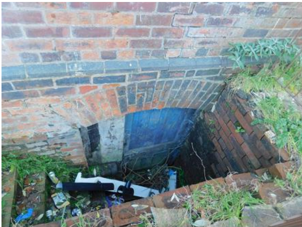
PHOTO 7 Entrance to Cellar
