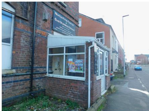
PHOTO 11 Eastern Elevation of Entrance
