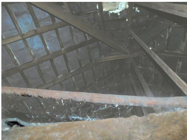
PHOTO 55 Underside of North-eastern Corner Roof
