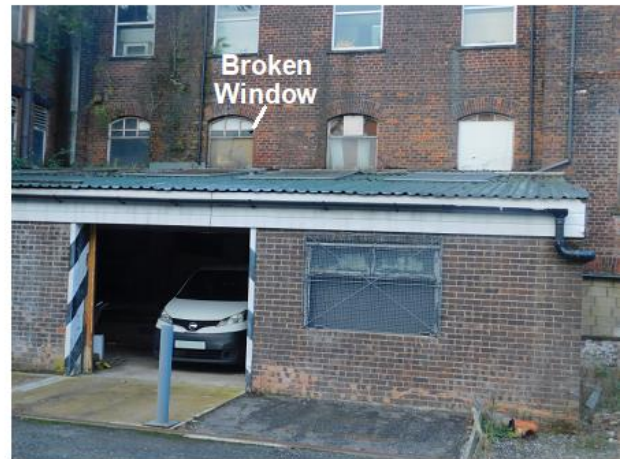
PHOTO 36 Southern Elevation of Shed
