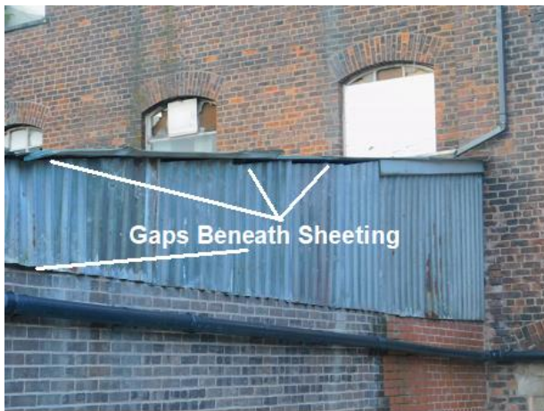
PHOTO 37 Upper Eastern Elevation of Shed
