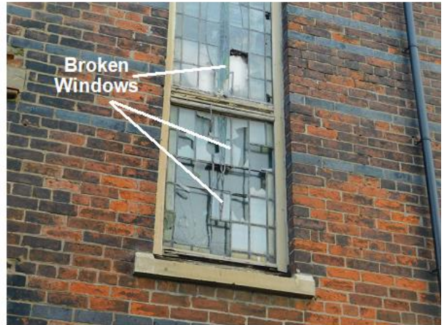
PHOTO 18 Central Western Elevation
