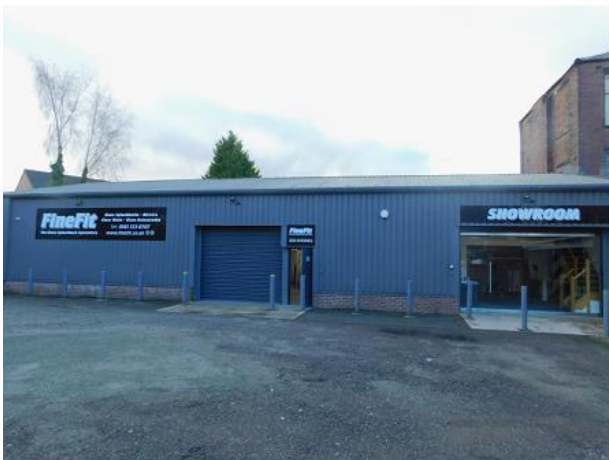
PHOTO 27 Eastern Elevation of Showroom
