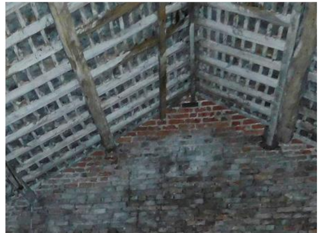
PHOTO 48 Underside of South-western Stores Roof
