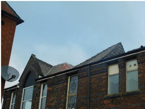
PHOTO 17 View of Upper Western Elevation
