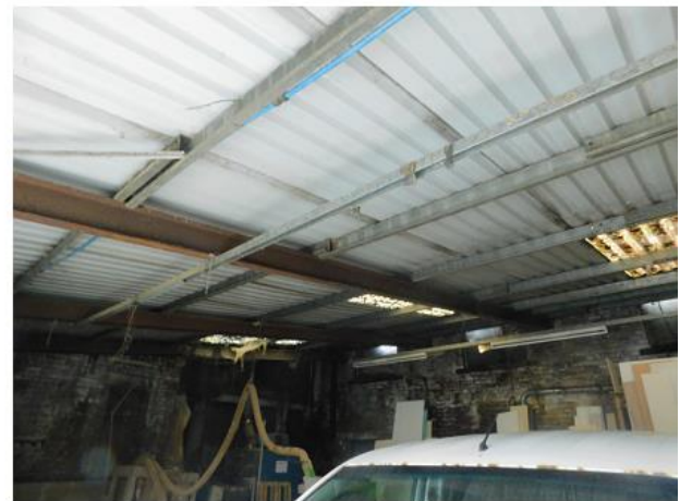
PHOTO 40 Underside of Shed Roof
