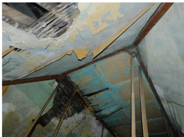
PHOTO 50 Underside of Office Void Roof
