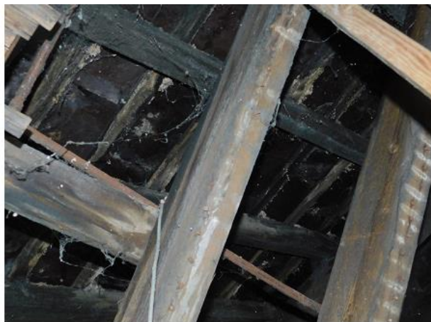
PHOTO 56 Underside of Eastern Roof Void
