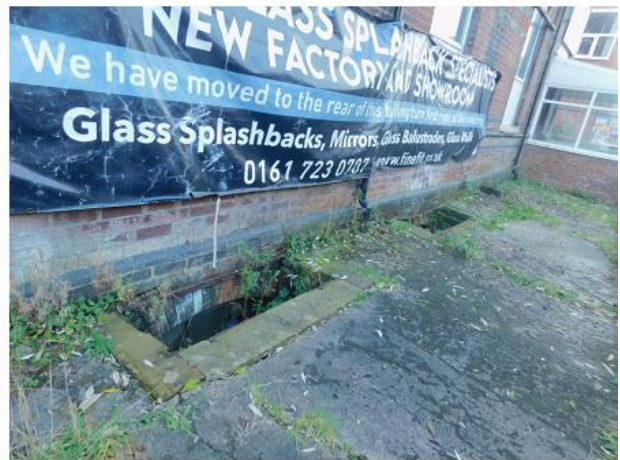
PHOTO 10 South-western Basement Vent
