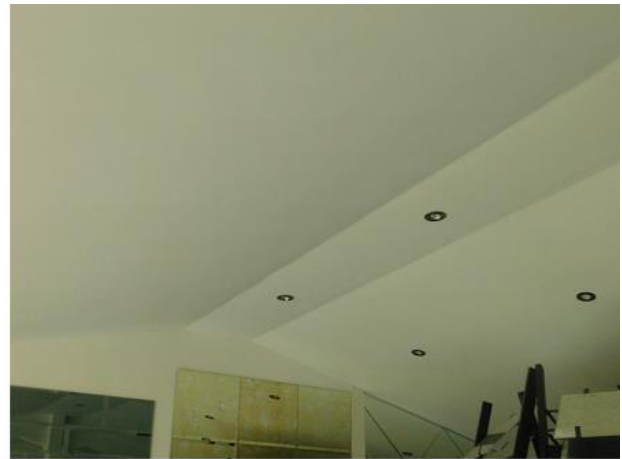
PHOTO 32 Underside of Showroom Office Roof
