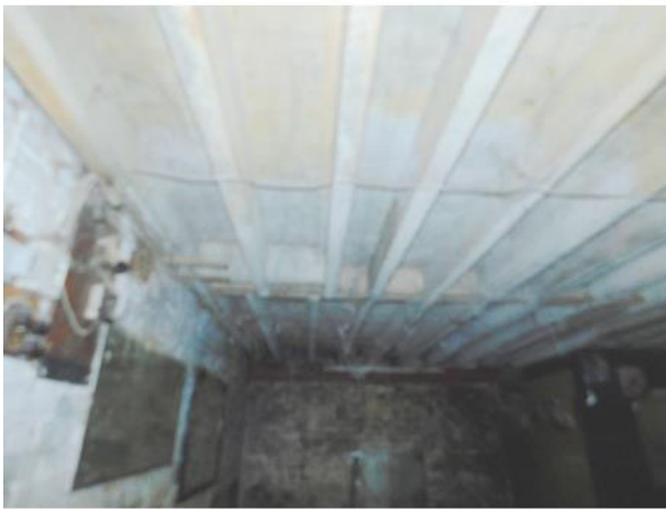
PHOTO 45 Western Basement Roof
