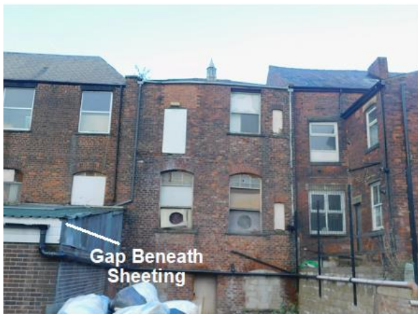
PHOTO 41 Central Southern Elevation of Main Building
