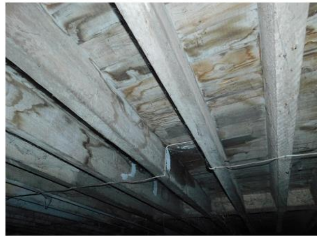
PHOTO 46 Eastern Basement Roof
