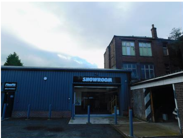
PHOTO 29 North-eastern Elevation of Showroom
