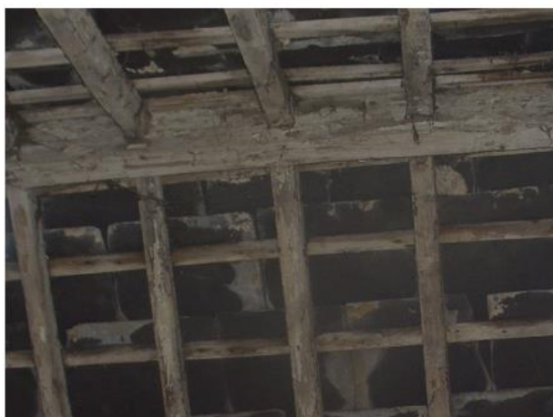
PHOTO 57 Underside of South-eastern Corner Roof
