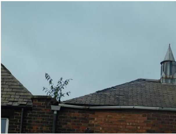
PHOTO 43 Part Upper Central Southern Roof
