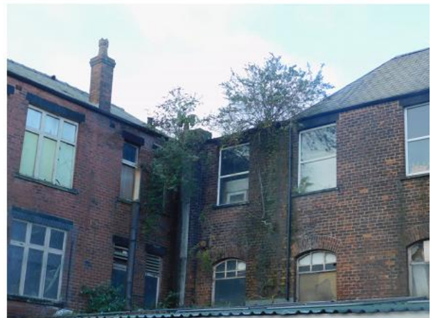
PHOTO 34 South-eastern View of Hipped Joint
