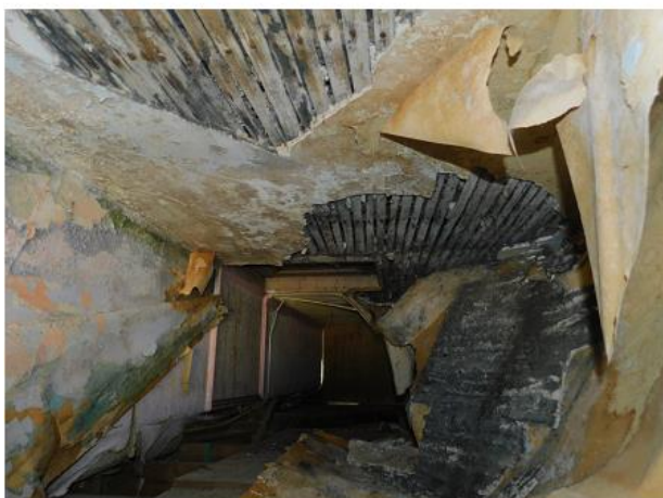
PHOTO 53 Underside of Typical Dormer Roof
