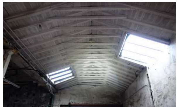
Timber clad roof area.
