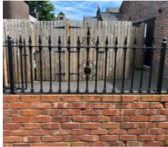
Image 08 – Existing boundary wall & railings to adjacent property (16 St Mary's Place).
