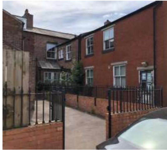
Image 07 – Existing boundary wall & railings to adjacent property (16 St Mary's Place).
