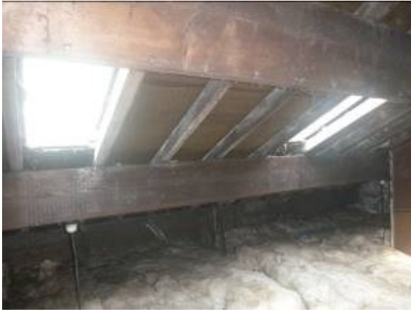
P9 No. 10 void showing roof felting and insulation
