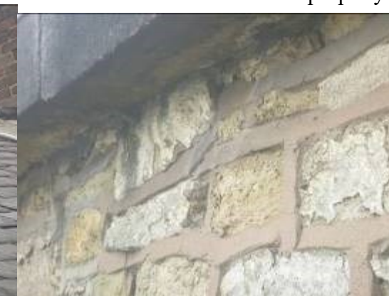
P6 Well-sealed eaves under stone gutters
