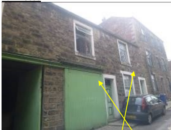
P1 Front (west) aspect, nos. 10, 12
