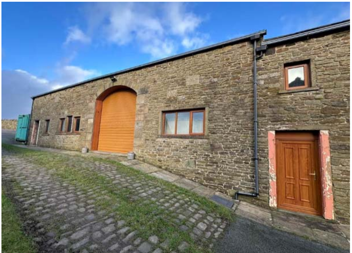
Cottage and barn attached to the house are probably early 19 th century
