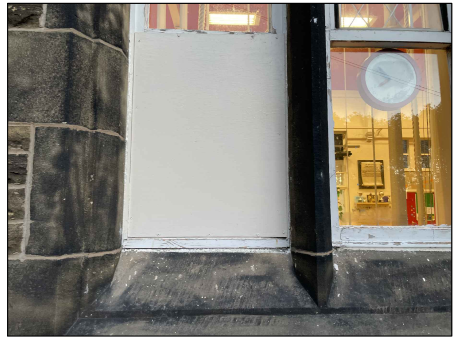
Image of stone window surrounds; the depth of which are to remain unchanged by the proposed window replacement.
