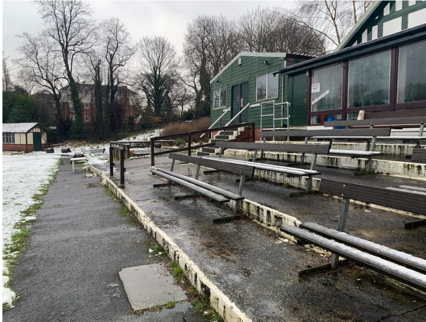
The crumbling seating area will be covered to create an elevated view over the pitch with new seating at the pitch side.
