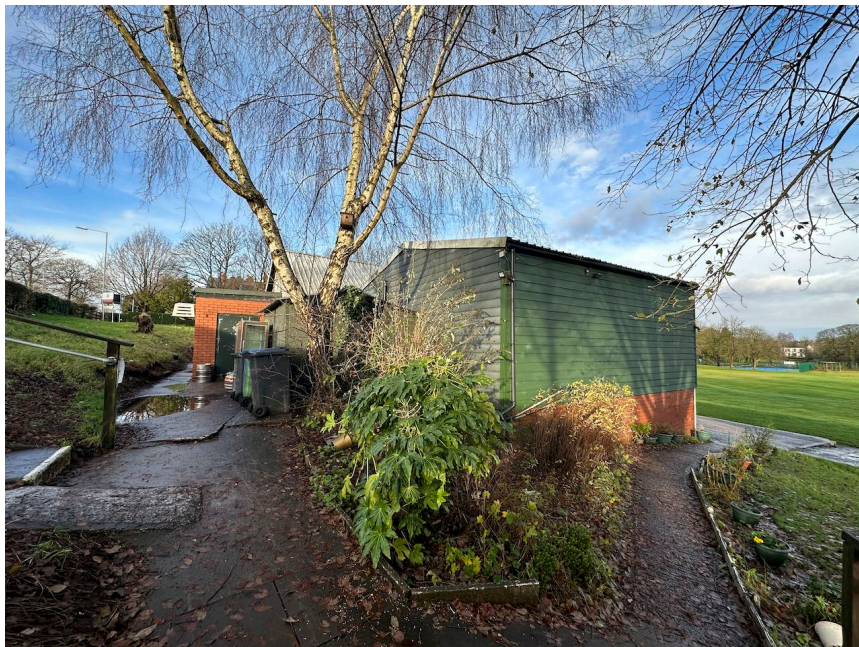
The rear of the club buildings that face Higher Lane. The changing rooms make up the green clad block and the removal of the birch tree, dilapidated concrete shed and bins to accommodate the extension will improve the visual asthetic of the area. The path will be relaid to improve accessibility.
