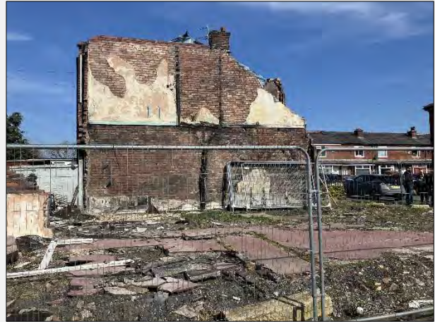
Plate 6: From south facing north 106 and 104 demolished, 102 wall in shot
