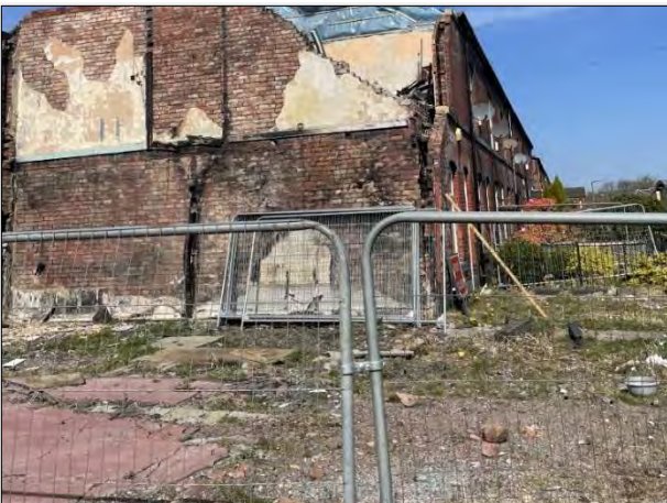
Plate 9: From southeast facing northwest
