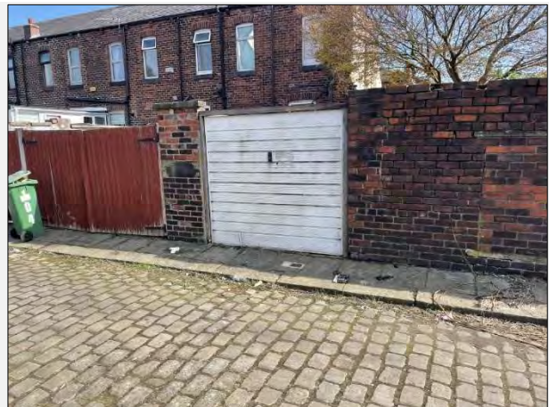
Plate 10: From west facing east
