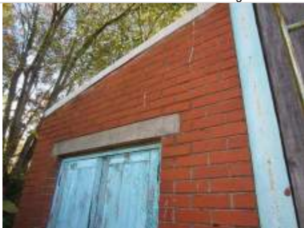
Photo 35: West elevation of Building 15
