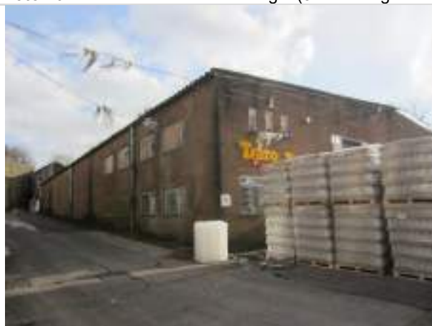
Photo 22: North and west elevation of Building 8
