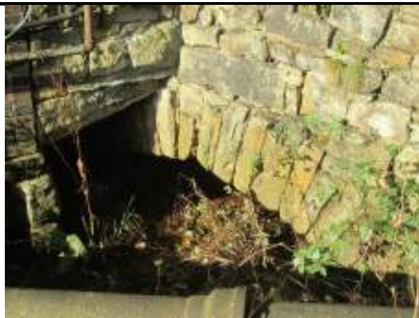
Photo 38: Culvert entrance near weir
