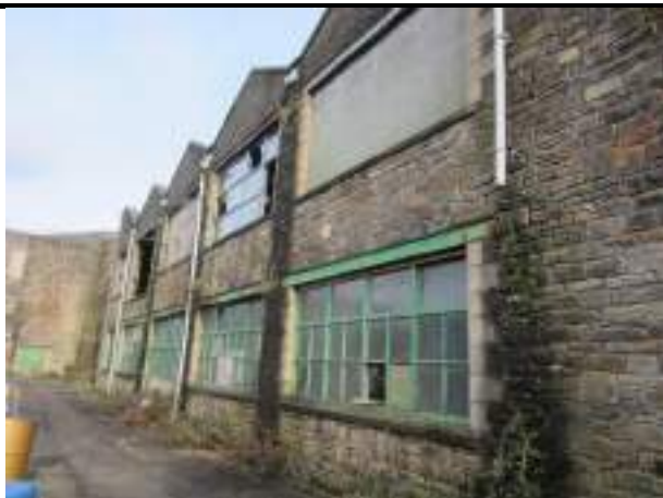
Photo 31: West elevation of Building 13
