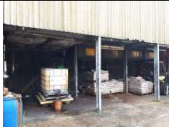
Solvent Filling room at Area 10
