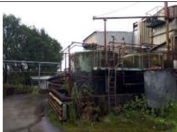
Solvent Filling room at Area 10
