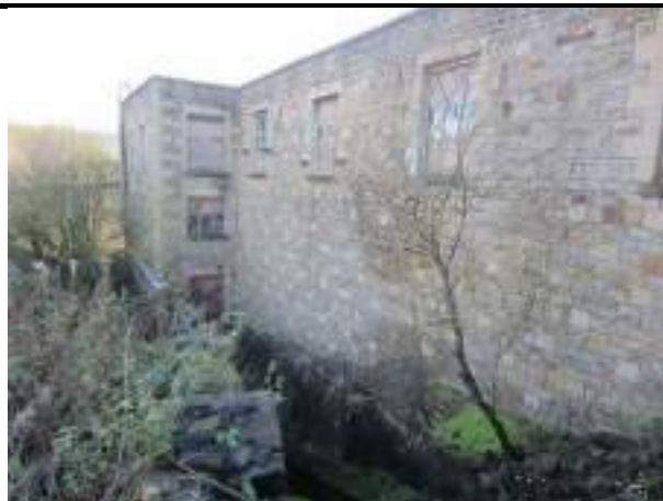
Photo 14: North elevation of Building 5a
