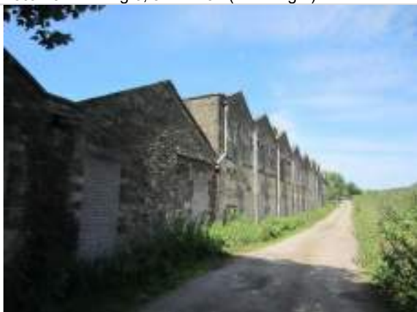
Photo 17: East elevation of Building 6 showing tightly sealed window apertures
