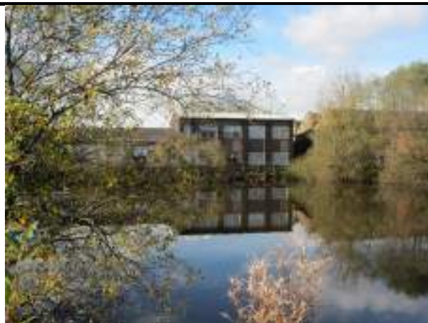
Photo 8: East elevation of Building 4 and lodge (Pond 1)
