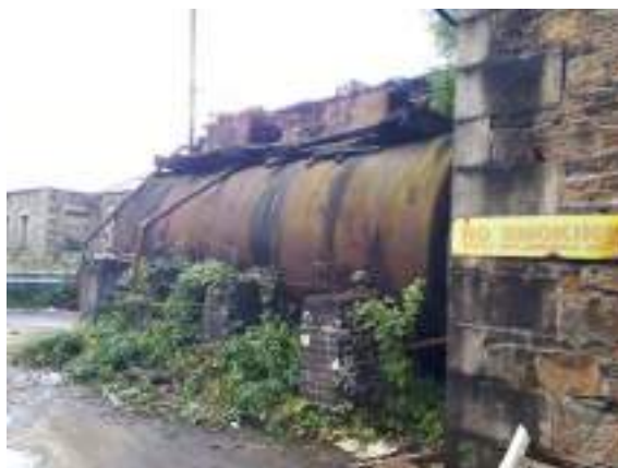
Additional 'hot' bitumen product tank near top of dam (west of Area 8)
