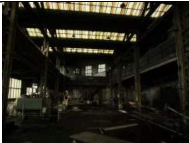
Photo 32: Interior of Building 13
