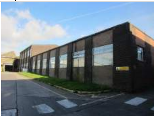
Photo 9: West and south elevation of Building 4
