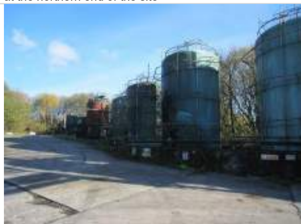
Photo 9: Hard-standing around the operational Tetrosyl site
