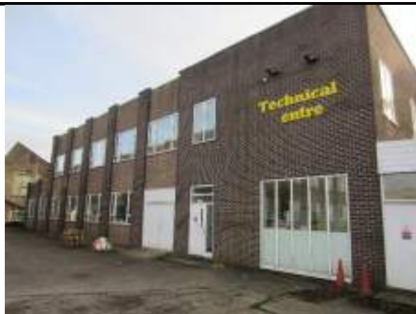
Photo 26: North and west elevation of Building 10
