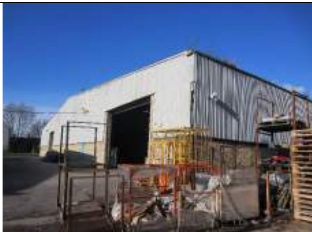
Photo 1: South and east elevation of Building 1
