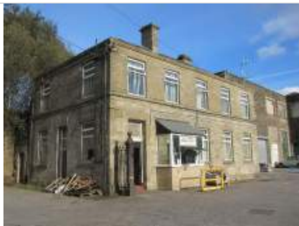
Photo 24: West and south elevation of Building 9
