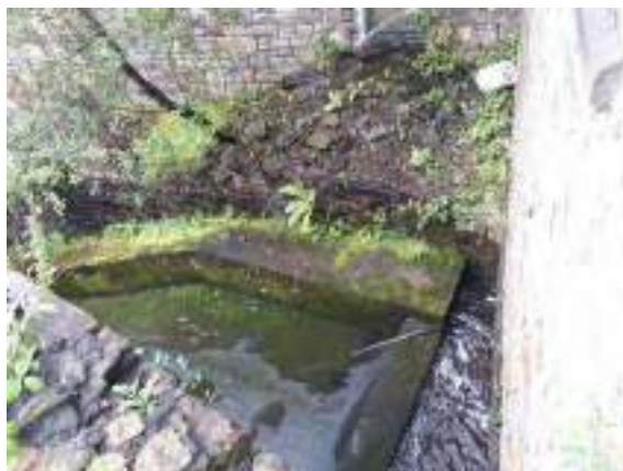
Inlet to culvert (Sample Analysis 17-65246; sample ref: SW-DU)
