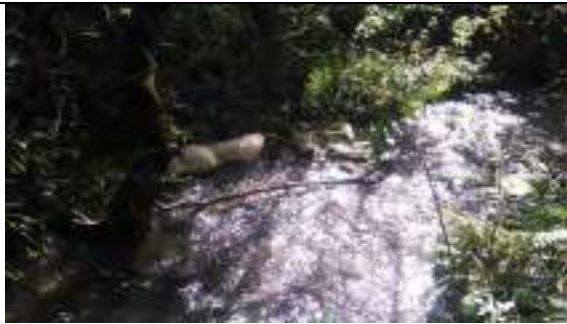
Off-site outfall to culvert (Sample Analysis 17-65246; sample ref: SW-DS)
