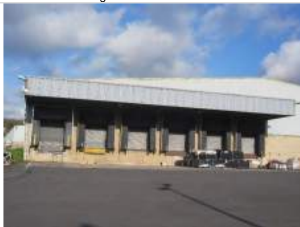
Photo 4: South elevation of Building 2
