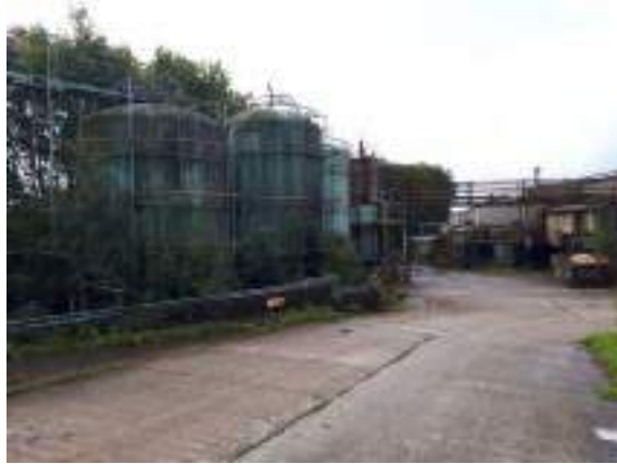
Tank Farm at area 11
