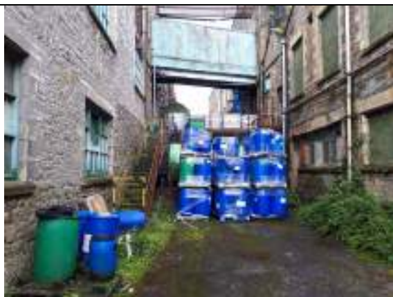
View towards area 6 numerous unbanded drum / IBC stores restrict access
