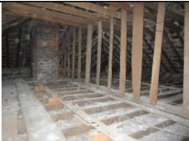
Photo 25: Roof void at Building 9
