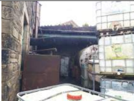
Oil AST in Area 3
