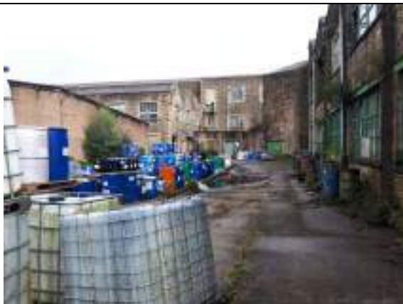
Drum Store in Area 2
