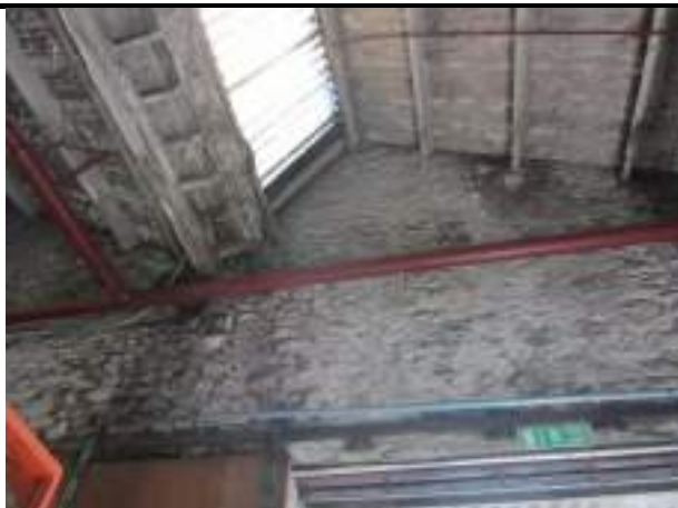
Photo 7: Interior of Building 3 showing sarking, north lights and exposed stone walls
