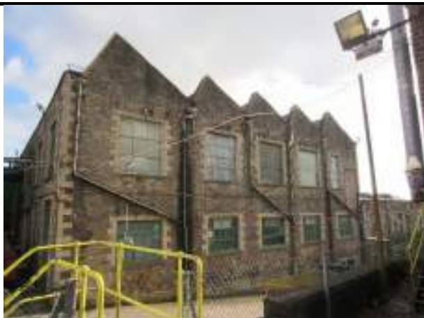
Photo 19: West elevation of Building 7
