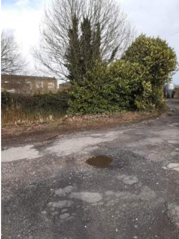
Pic 3 – JK area view to farm entrance
