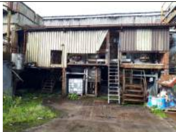
Solvent Filling room at Area 10
