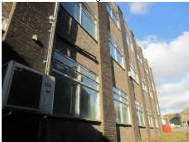
Photo 27: East elevation of Building 11b
