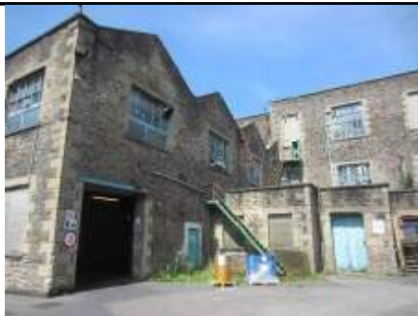
Photo 20: South elevation of Building 7 (5b in background)
