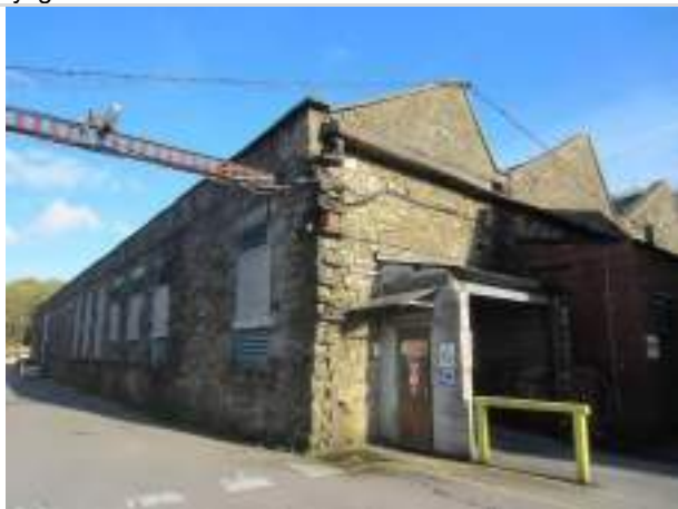
Photo 5: West and south elevation of Building 3
