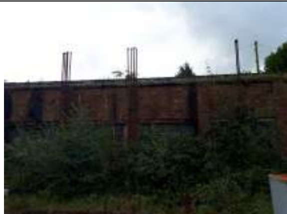
Assumed vents for USTs in Area 1
