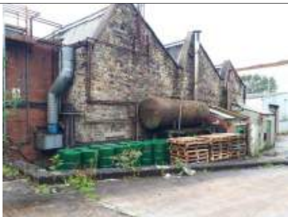
Solvent Filling room at Area 10
