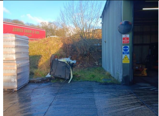
Photograph 6: View from southwest facing north, showing change in elevation on site and proposed kiosk location.
