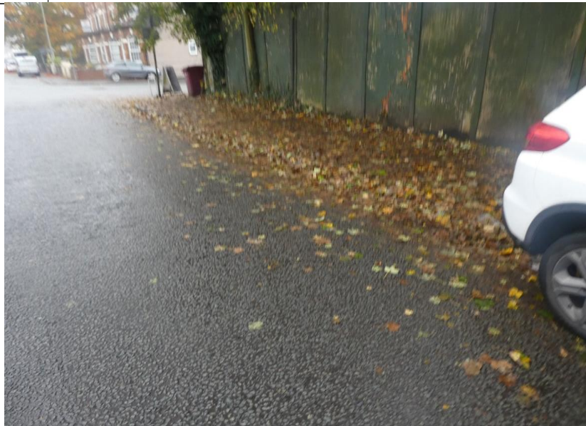
Photograph 76. Road surfacing in reasonable condition
