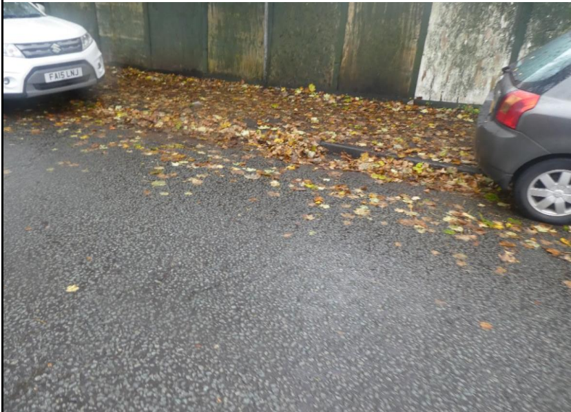
Photograph 75. Road surfacing in reasonable condition
