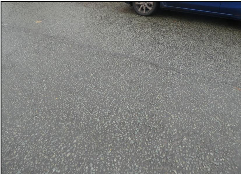
Photograph 57 Surfacing in reasonable condition.
