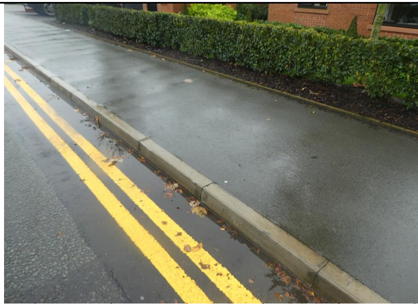
Photograph 54. Footpath in reasonable condition
