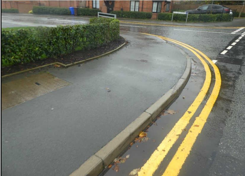
Photograph 55. Footpath in reasonable condition
