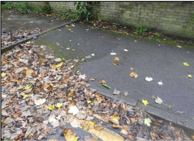
Photograph 13. Tarmacadam surfacing to the footpath
