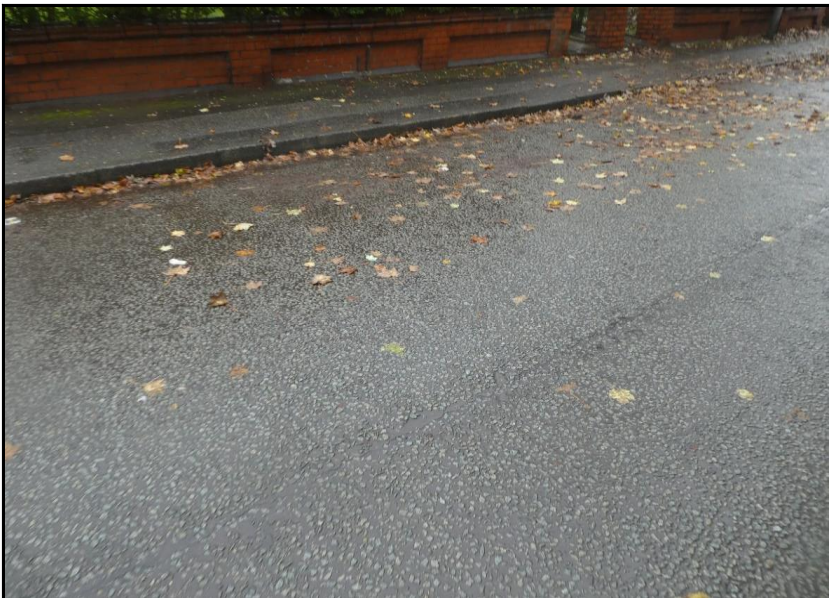
Photograph 73. Road surfacing in reasonable condition
