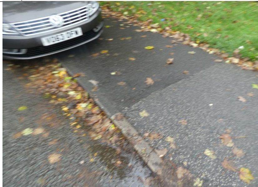
Photograph 72. Footpath in reasonable condition
