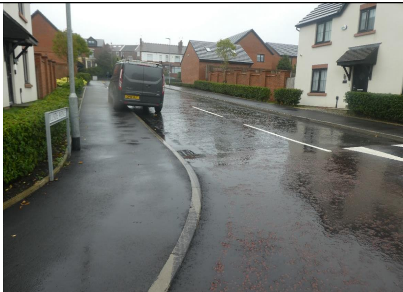
Photograph 2. Recently formed roadway and footpath surfacing
