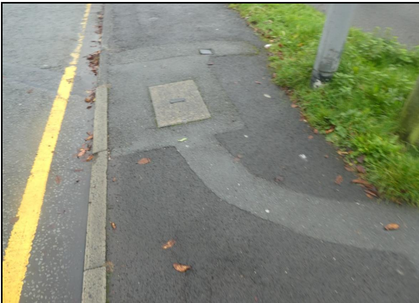
Photograph 65. Localised reinstament to footpath
