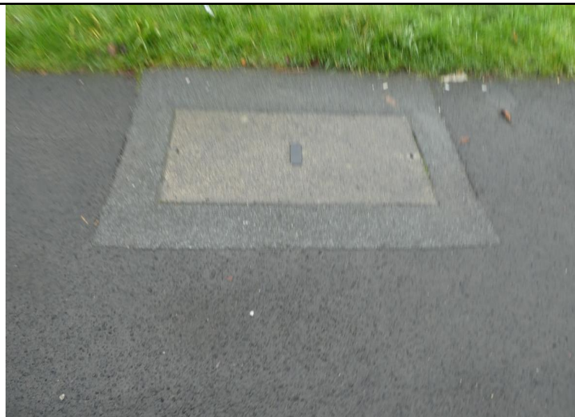
Photograph 66. Localised reinstament to footpath
