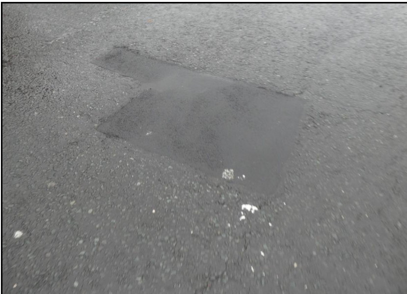
Photograph 85. Localised reinstatement of road surfacing.
