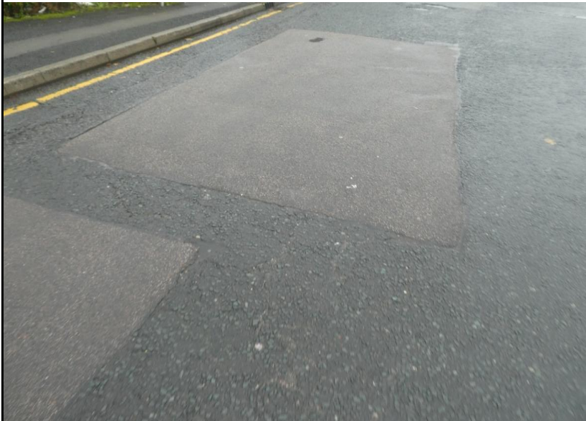
Photograph 87. Reinstatement of road surfacing.
