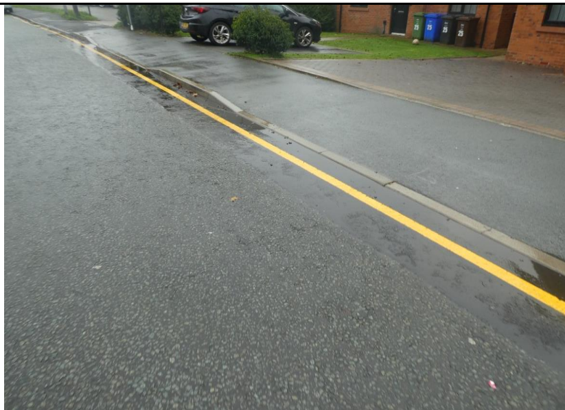
Photograph 58. Surfacing in reasonable condition.
