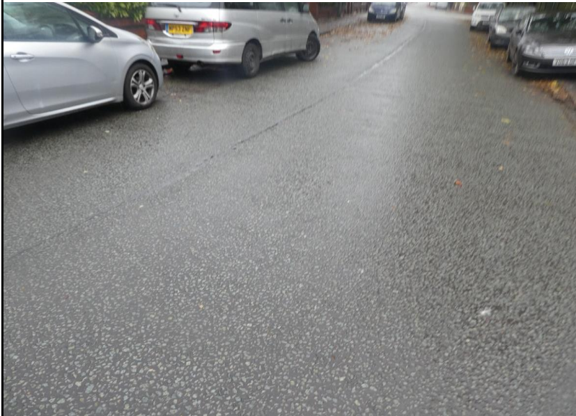
Photograph 71. Road surfacing in reasonable condition
