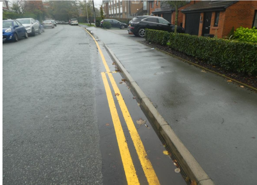
Photograph 56. Footpath in reasonable condition
