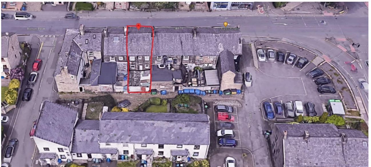
Figure 9 | Street Scene along Pilkington Street | Google Image
