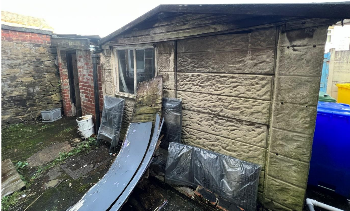
Figure 7 | Out-building elevation facing internal yard
