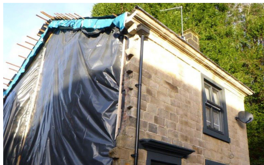
Stone detailing at 6 East View Window surrounds, gutter cornice and moulded cornice above front door
