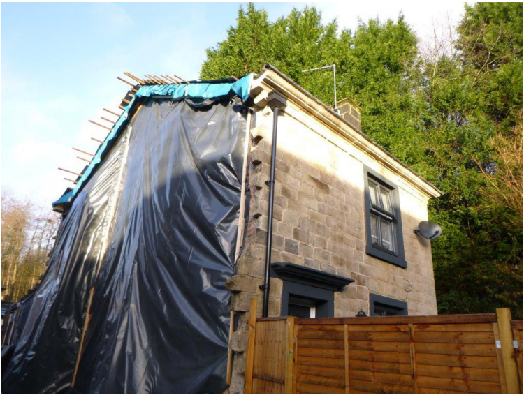
6 East View in December 2022
