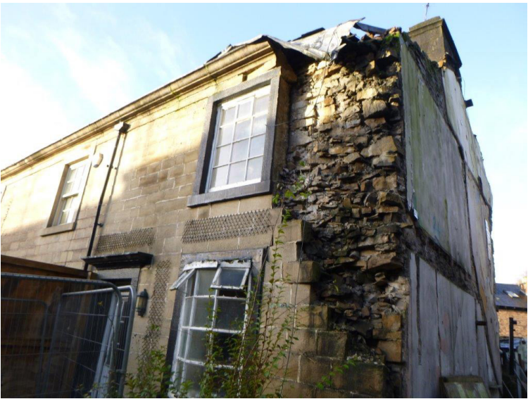
4 East View in December 2022
