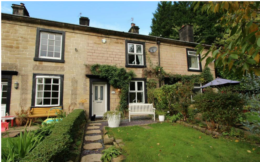
Figure 1.3: Front elevation 5 East View prior to explosion (2019)
