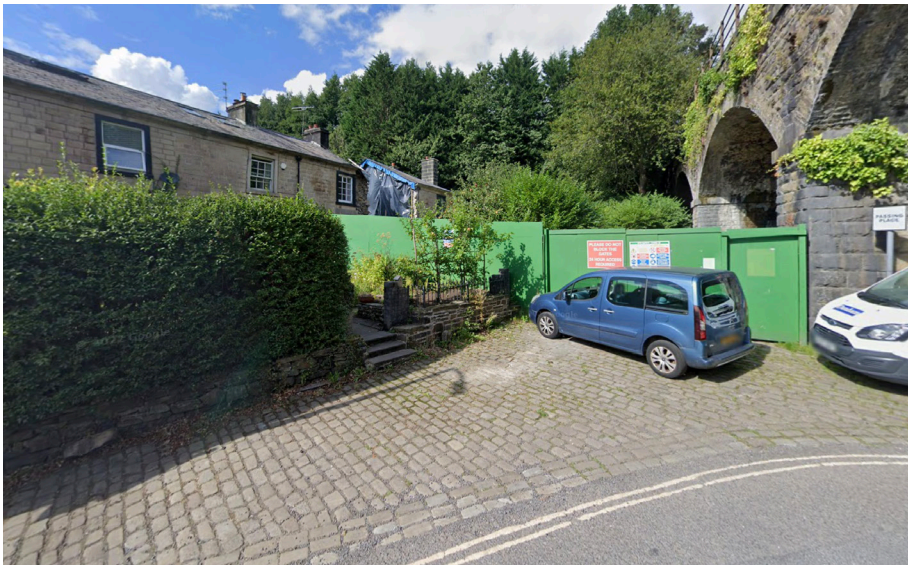
Figure 1.1: View from Waterside Road
