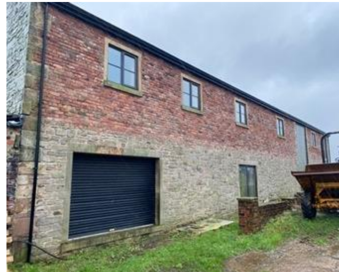
Fig. 10, Rear elevation of barn
