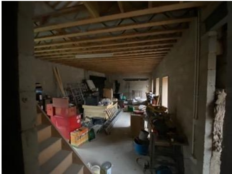
Fig. 11, Ground floor of barn
