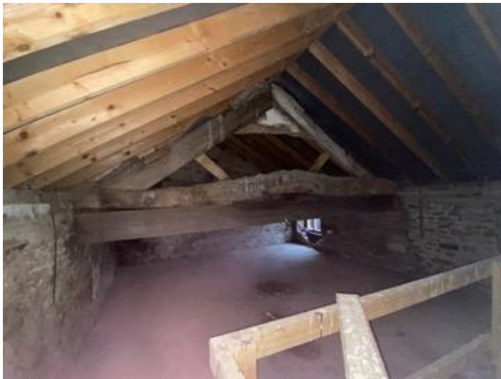
Fig. 8, Former hayloft to stables with truss
