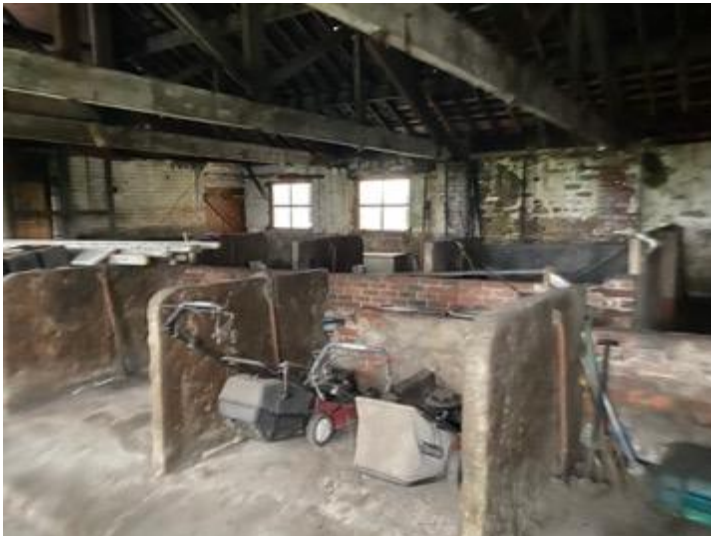
Fig. 16, Internal view of Shippen
