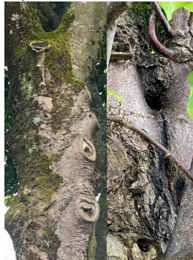
Photograph 10: Pruning cut holes and knot holes on T2
