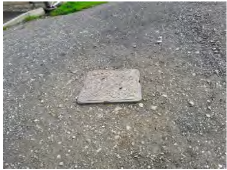
Photograph 5 (P5) View of drain on site.
