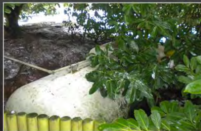
Tank in overgrowth
