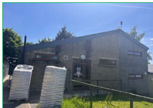
The building to the south
