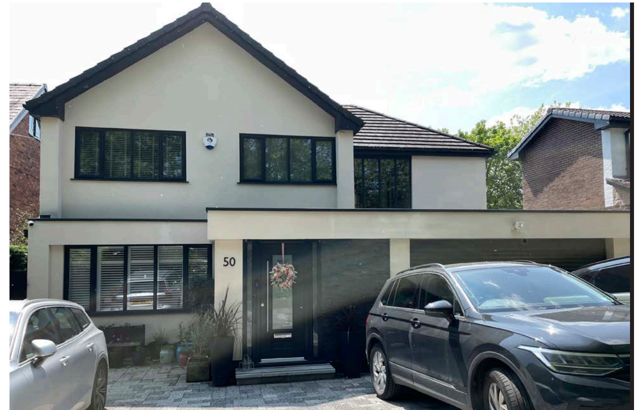
Above: Existing House - Front
