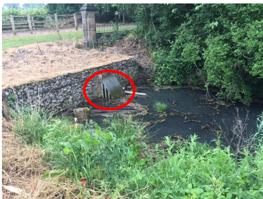
Plate 6: The end of Bealey's Goit near the proposed pitch area, note the start of the culverted section
