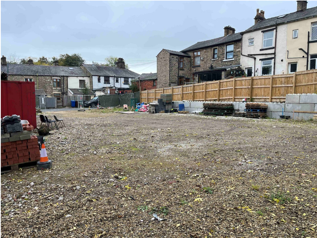
View to the south west corner
