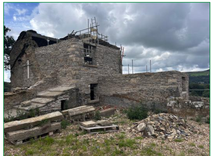
The northeast elevation of the structure
