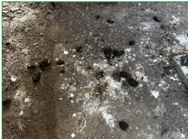
Showing barn owl pellets and droppings on the floor of the structure
