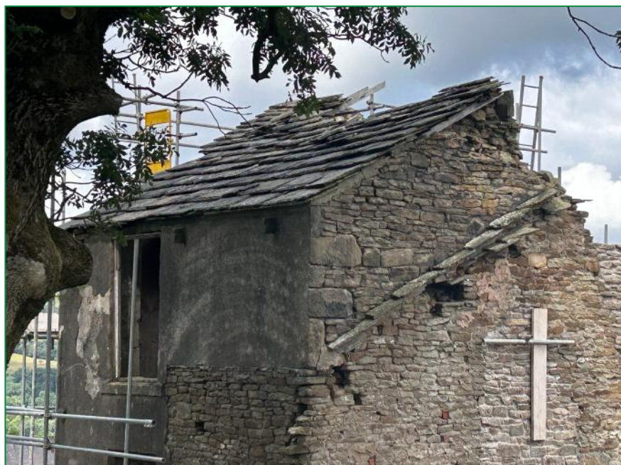
Showing southeast elevation of the structure and the partial roof on the south elevation.
