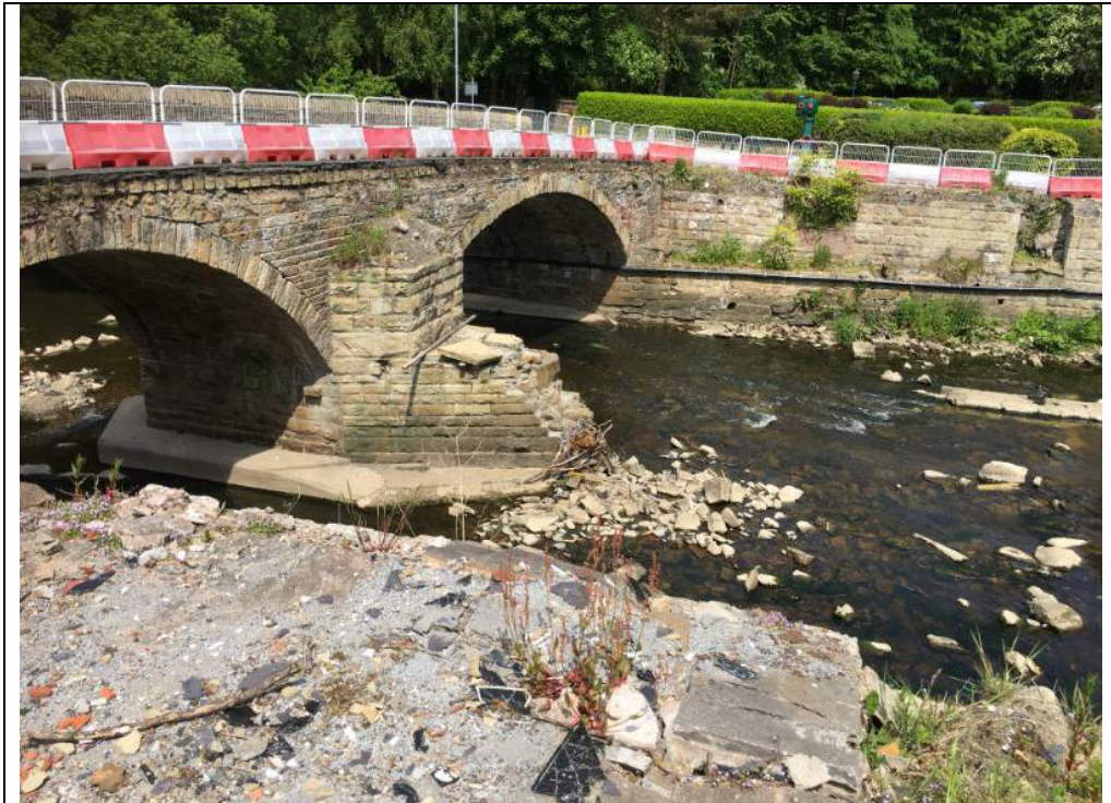
Figure 3: Kay Street Bridge viewed from proposed site
