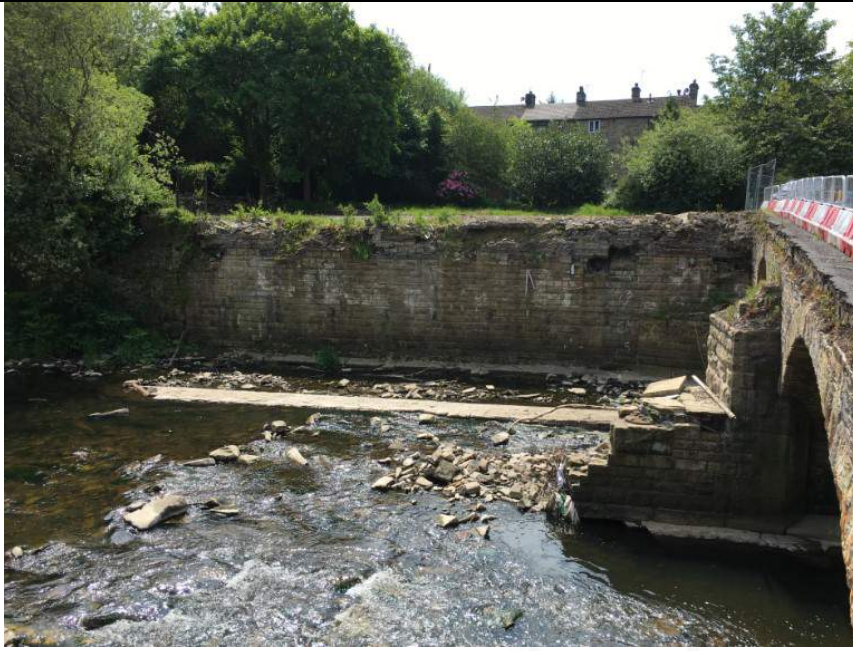
Development site looking from opposite bank
