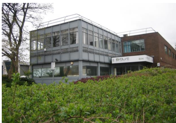
Figure 2: View of Link House from the south, looking northwards.
