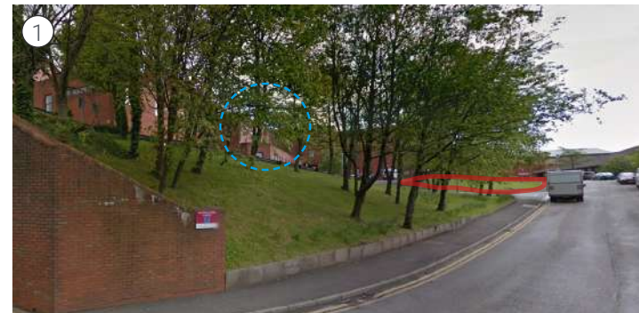
Primary Approach View from Hospital circulation road
