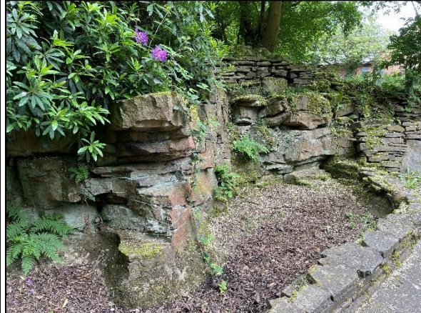
Figure 37: Further areas of rock to the southeast.
