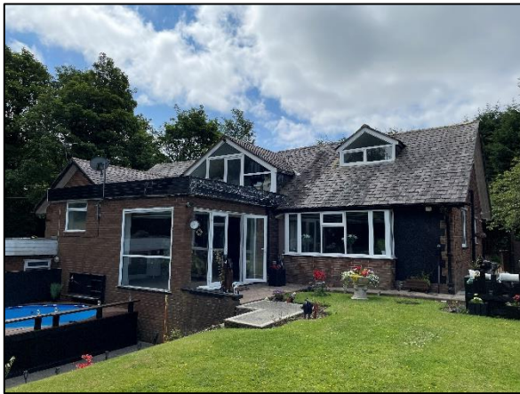
Figure 16: The northern elevation of the building.
