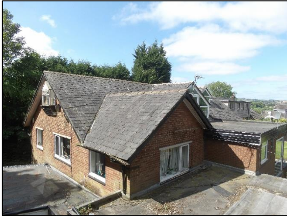
Figure 24: The roof of the building.
