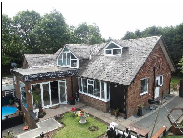
Figure 9: The property, viewed from the northwest.
