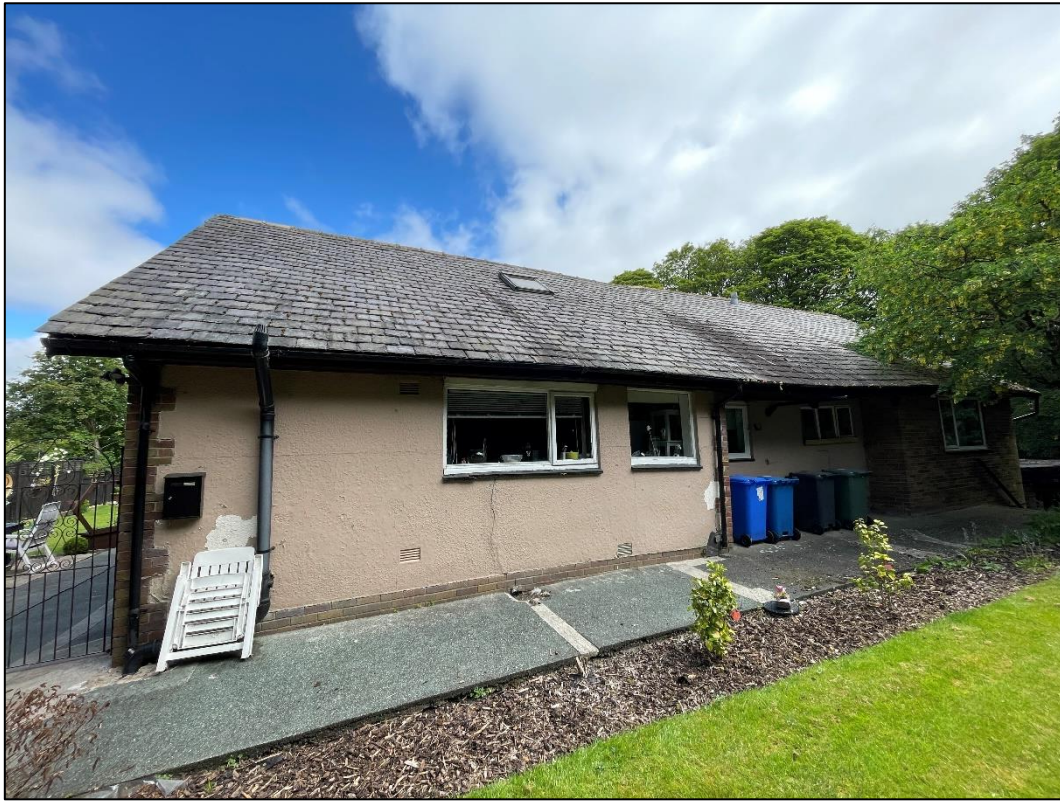
Figure 15: The southern elevation of the building.
