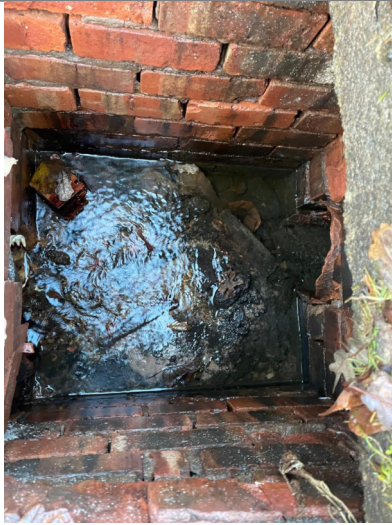
Manhole / Access Point: MH01 Internal
