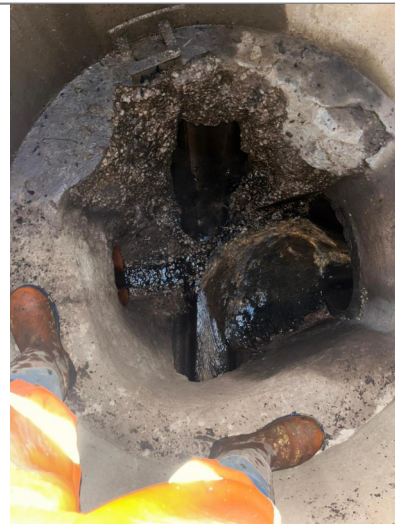
Manhole / Access Point: MH03 Internal
