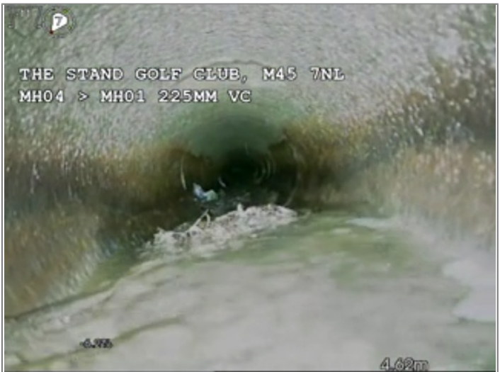
Roots mass 20% cross-sectional area loss
