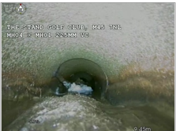
Roots mass 50% cross-sectional area loss
