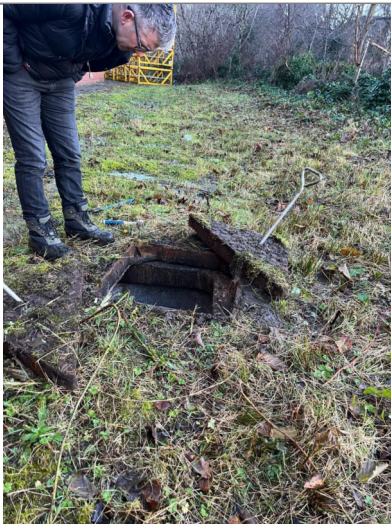
Manhole / Access Point: MH03 Location
