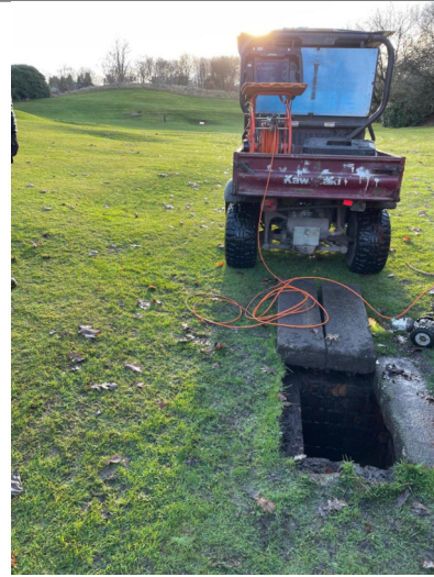
Manhole / Access Point: MH04 Location
