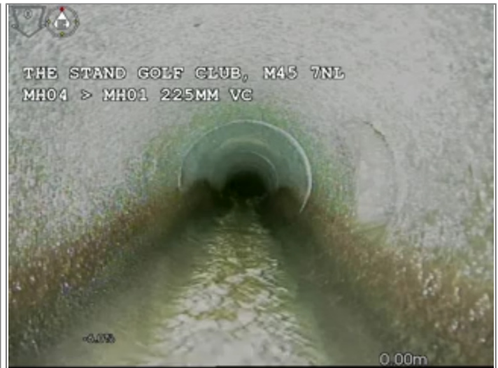
Water level 5% height/diameter
