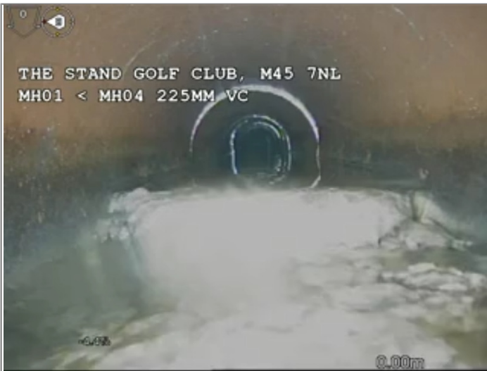
Start node type, Manhole, reference MH01
