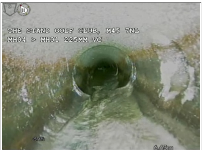
Junction at 03 o'clock, diameter 100mm
