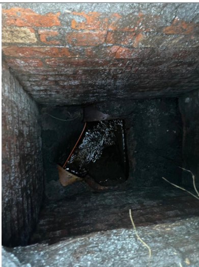
Manhole / Access Point: MH02 Internal
