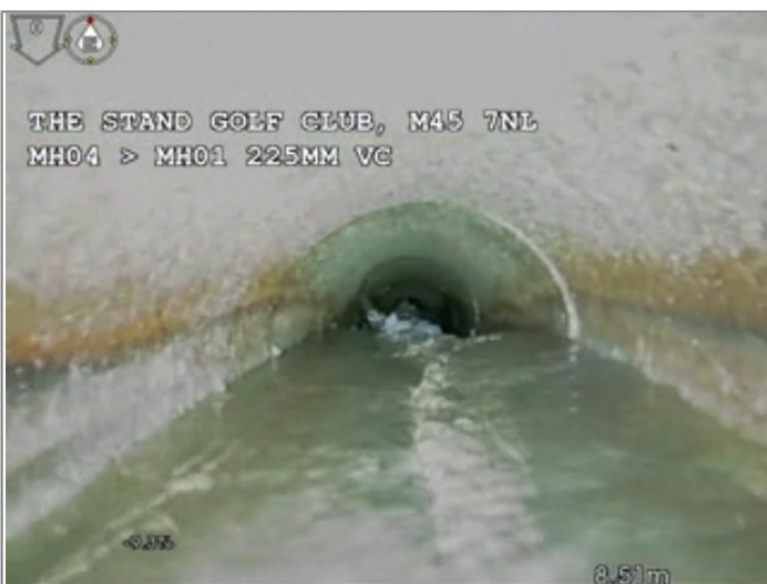
Water level 40% height/diameter
