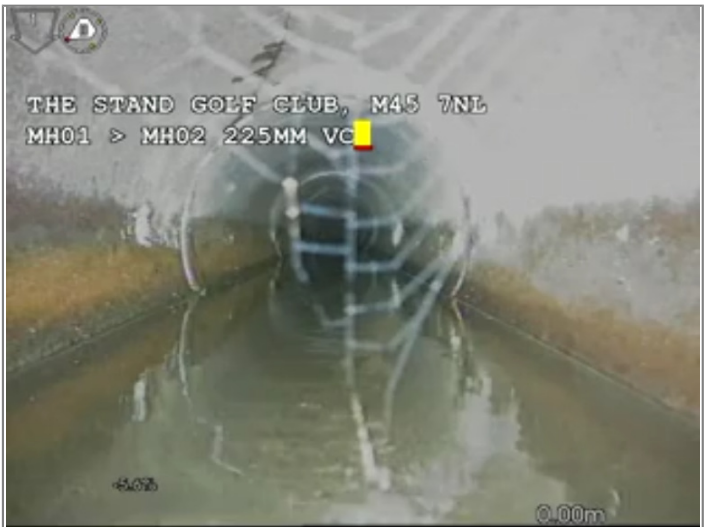
Water level 10% height/diameter
