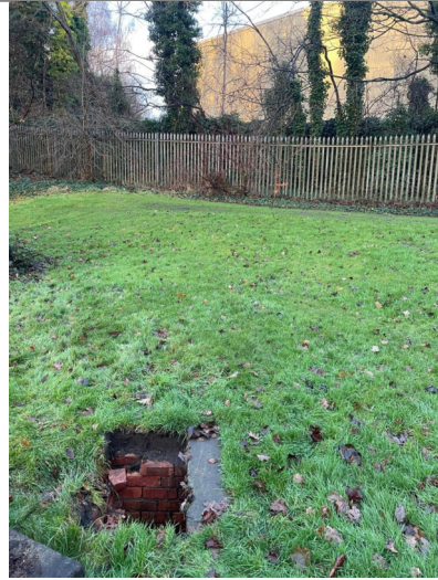
Manhole / Access Point: MH01 Location
