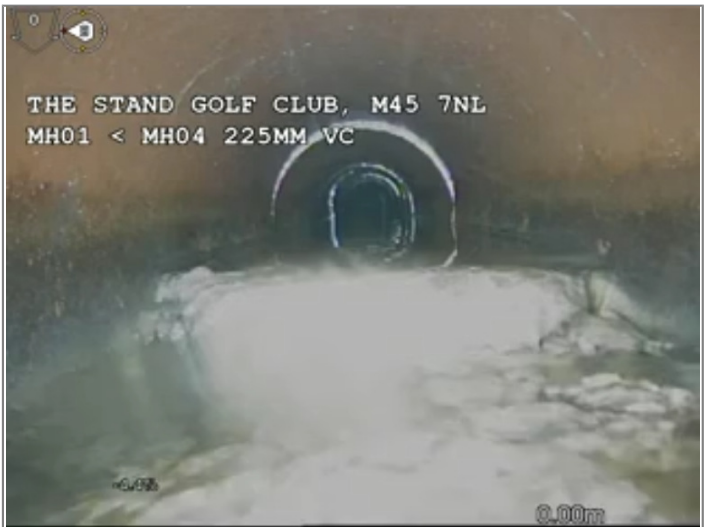
Water level 20% height/diameter
