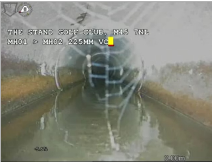
Start node type, Manhole, reference MH01
