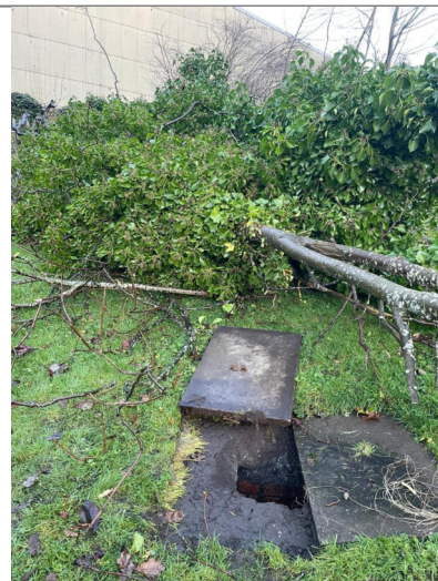
Manhole / Access Point: MH02 Location
