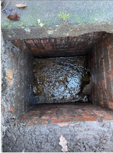
Manhole / Access Point: MH04 Internal
