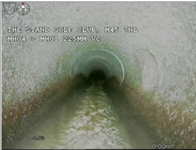
Start node type, Manhole, reference MH04
