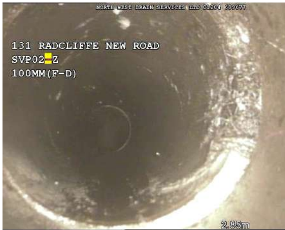
5, 00:00:28, 2.85 m Roots, fine at joint
