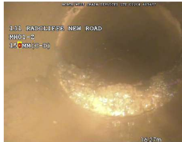
2, 00:01:46, 16.27 m Attached deposits, encrustation at joint from 3 o'clock to 9 o'clock, 30% cross-sectional area loss
