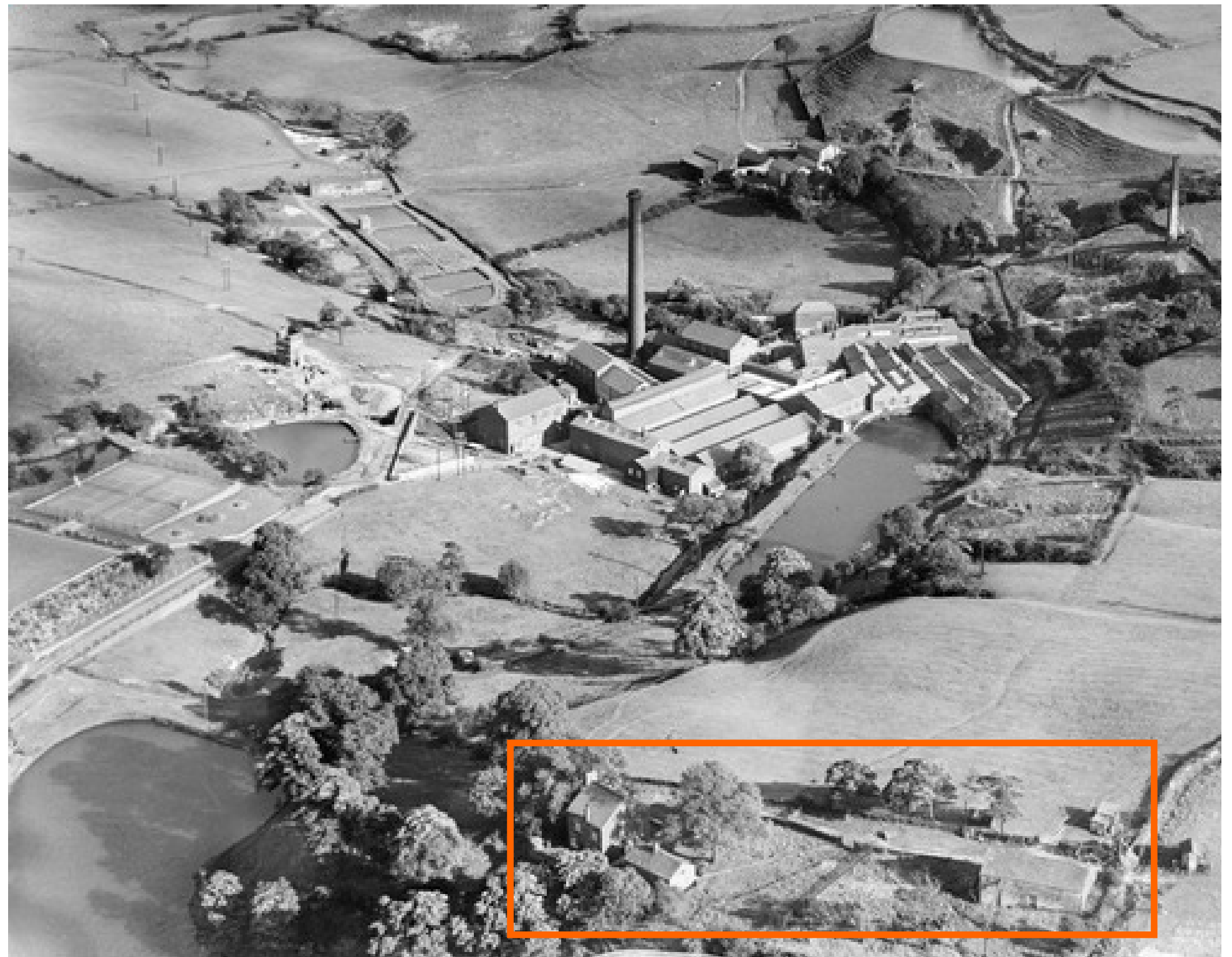
Historic photo of Two Brooks Bleach Works: 1929
