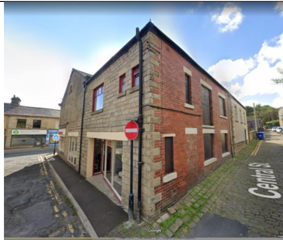
View of the rear along Central Street (Source: google Maps)
