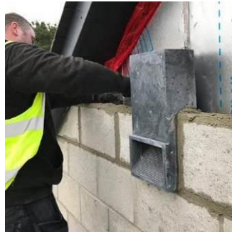
Green and Blue Bat Block/Brick in situ
