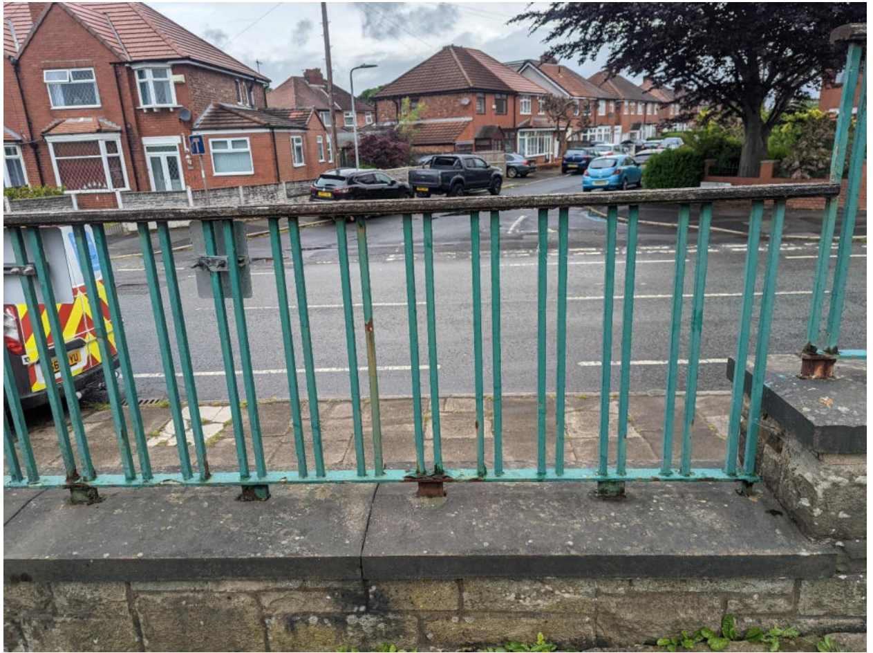
Plate 23: View of Heaton Park Reservoir Pumping Station (4) external handrail and balustrade, looking north-west.
