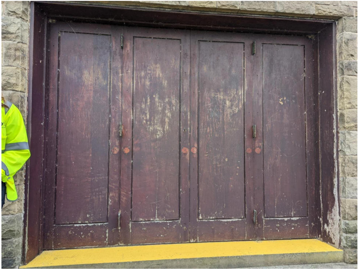
Plate 35: Exterior view of rear door of Heaton Park Reservoir Pumping Station (4).
