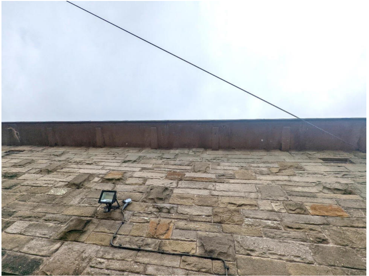
Plate 25: View of roof edge and external lighting on south-west elevation of Heaton Park Reservoir Pumping Station (4).
