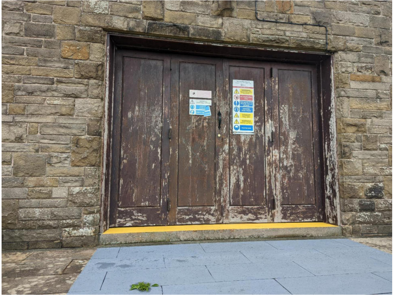
Plate 34: Exterior view of the front doors of Heaton Park Reservoir Pumping Station (4).
