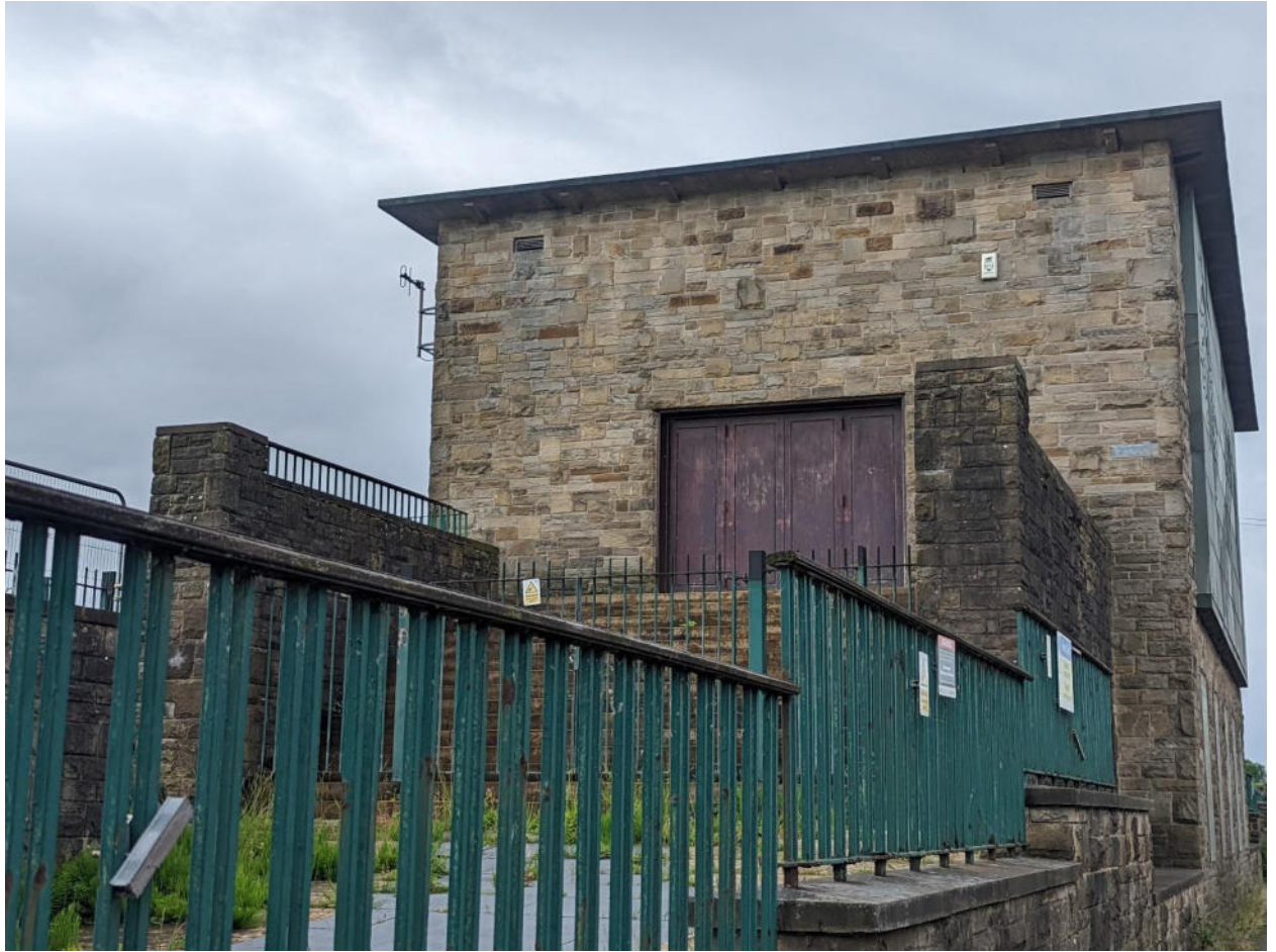
Plate 21: View of Heaton Park Reservoir Pumping Station (4) From Heywood Road, looking south-west.
