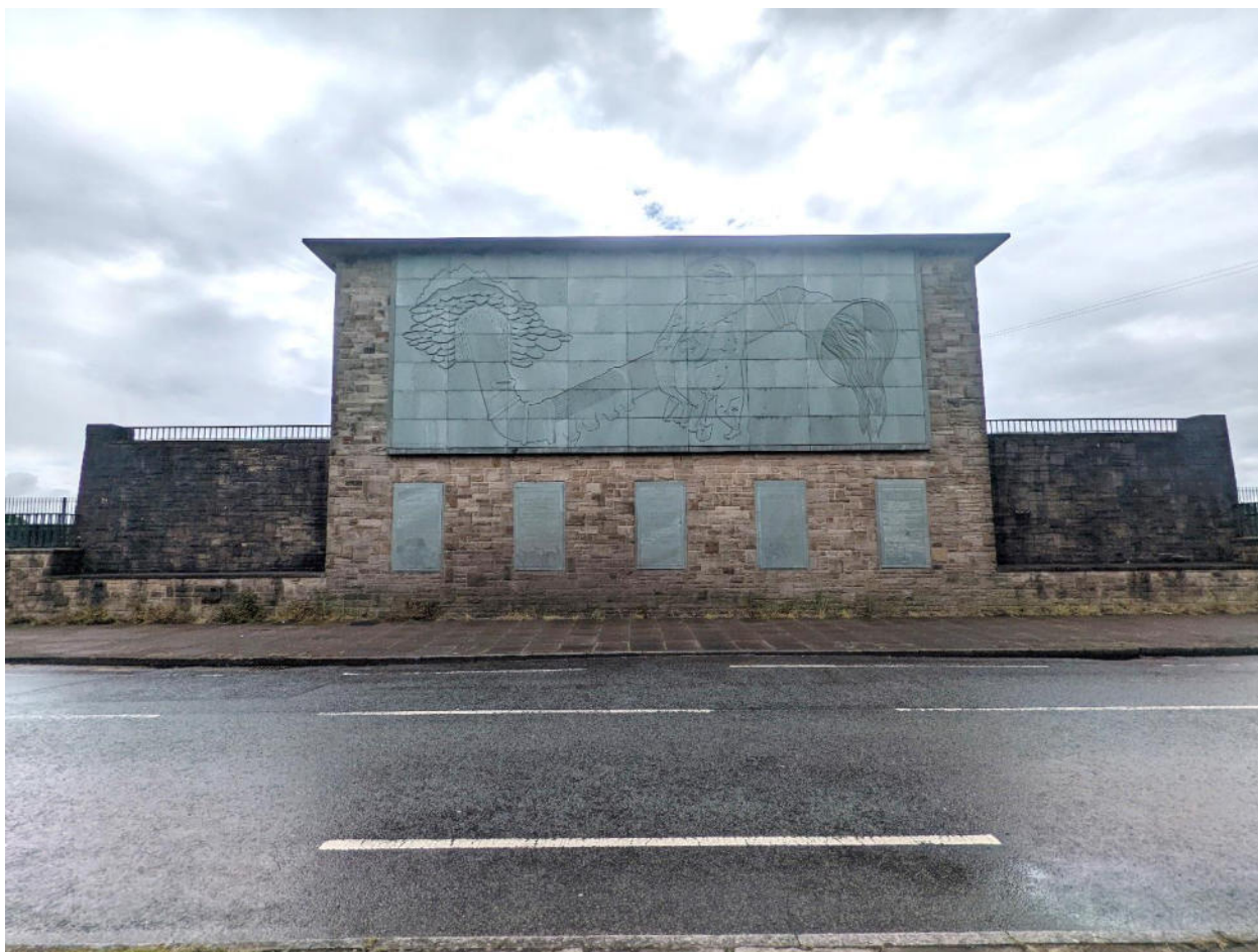
Plate 20: View of Heaton Park Reservoir Pumping Station (4) From Heywood Road, looking south-east.
