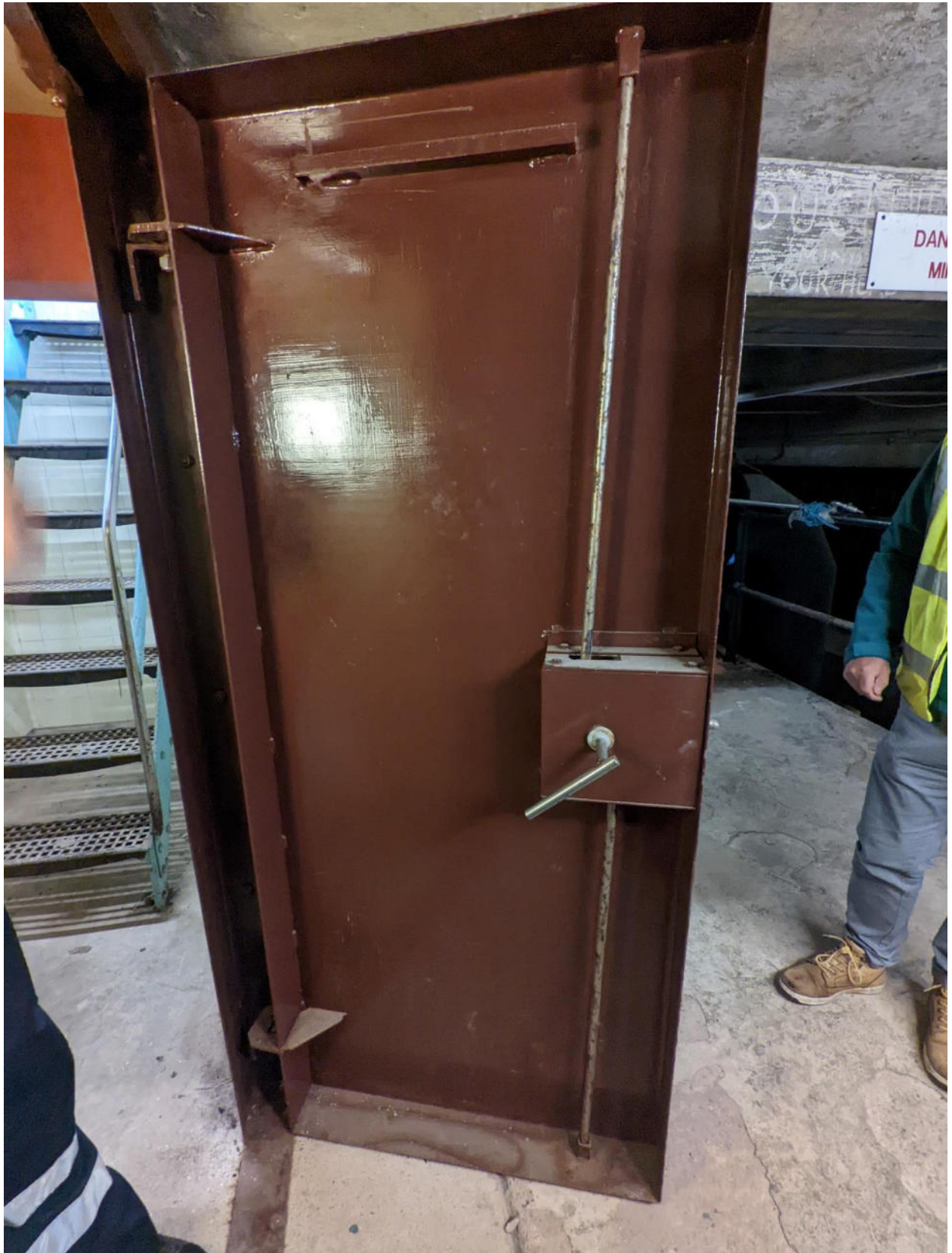
Plate 32: View of basement door of Heaton Park Reservoir Pumping Station (4).
