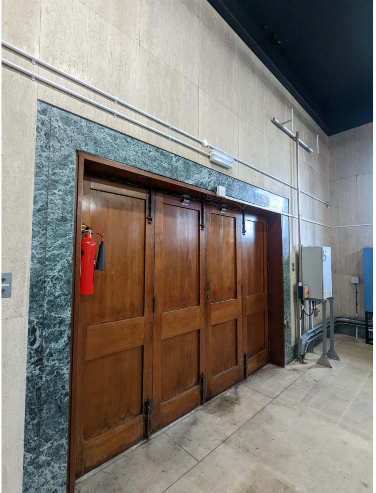
Plate 30: View of interior of rear door of Heaton Park Reservoir Pumping Station (4).
