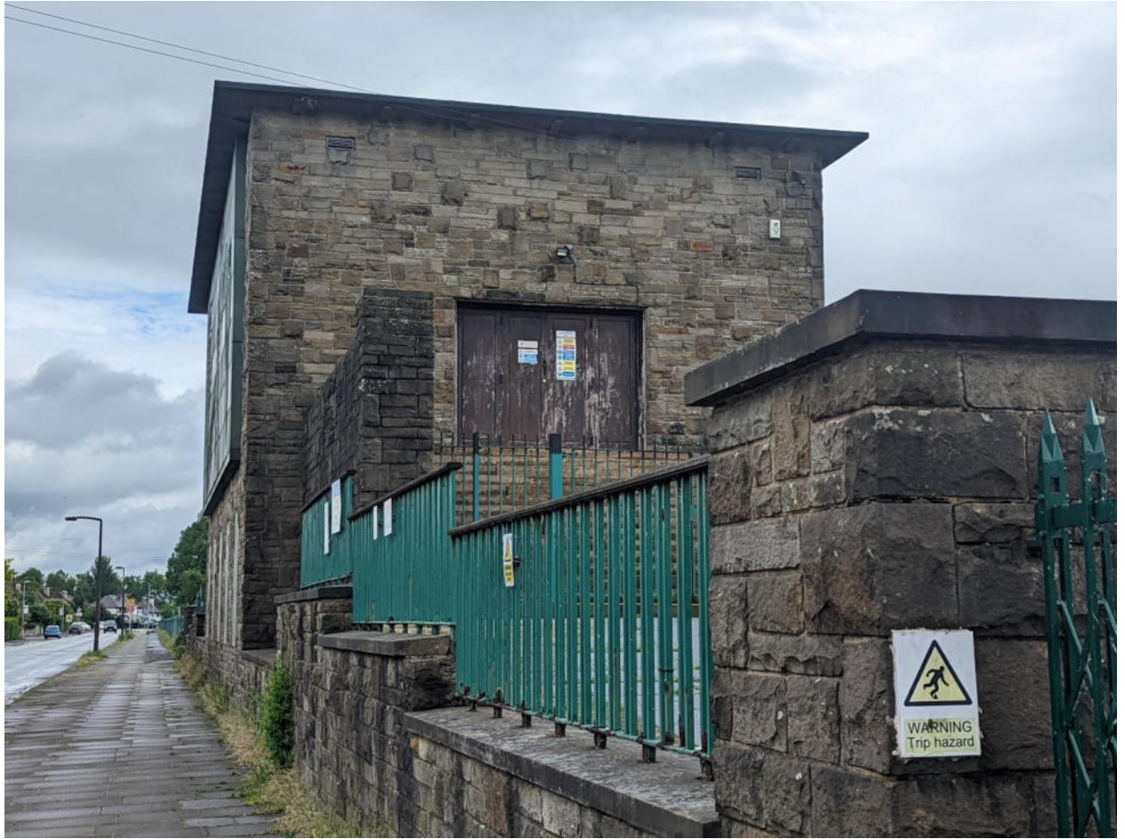
Plate 22: View of Heaton Park Reservoir Pumping Station (4) From Heywood Road, looking north-west.
