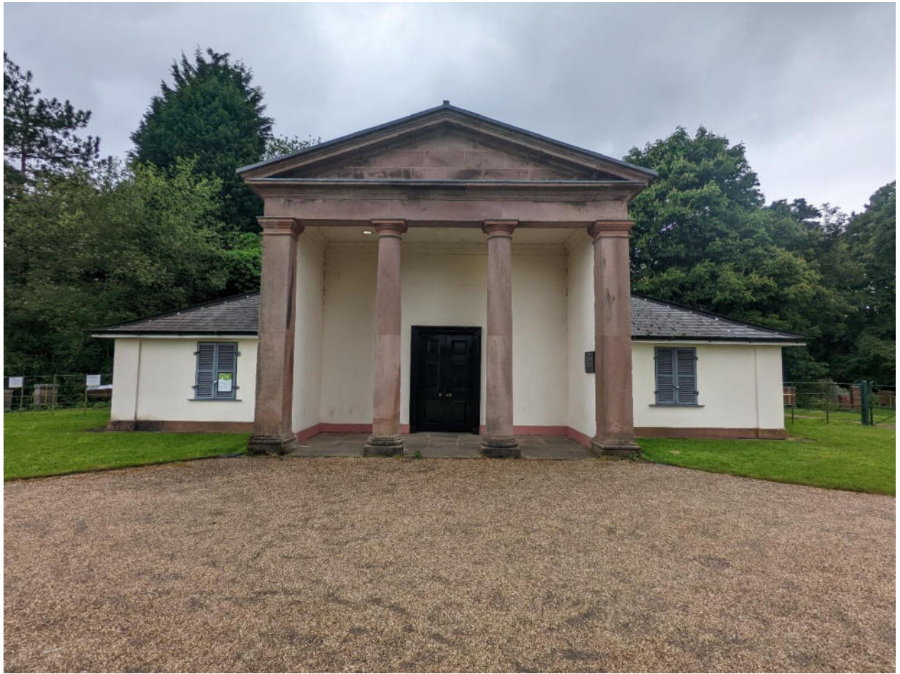
Plate 37: View of Dower House Cottage (1) towards Heaton Park Reservoir Pumping Station (4), looking north-west.
