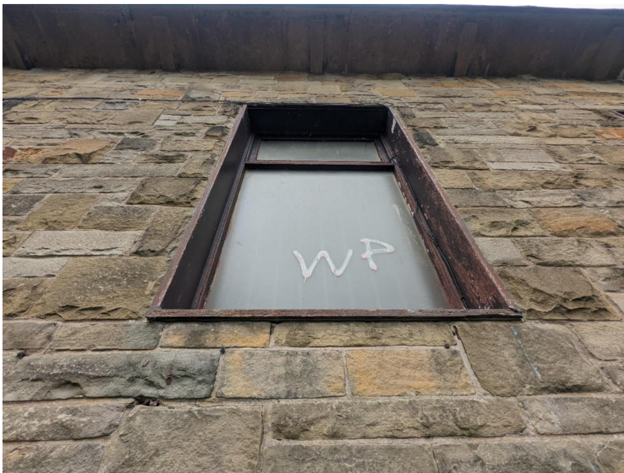
Plate 24: View external window frame on south-east elevation of Heaton Park Reservoir Pumping Station (4).
