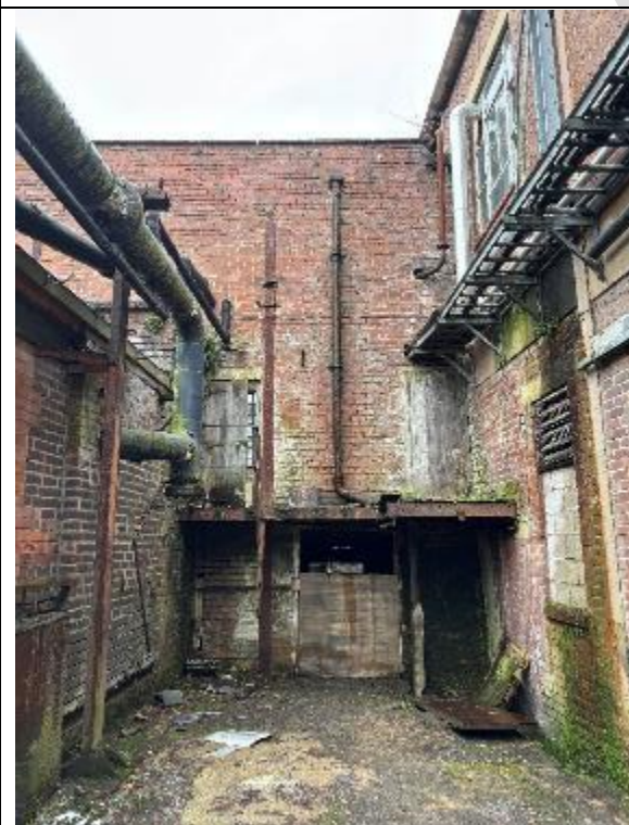
Photograph 11: View of the western area of the buildings.
