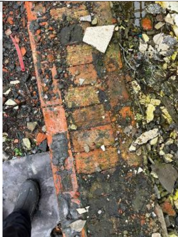
Photograph 16: View of exposed brickwork which shows there are no internal cavities within the brick walls.
