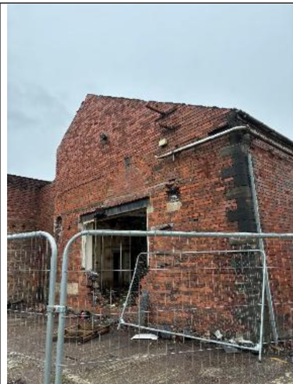
Photograph 5: View of the southeastern elevation (PRF2).
