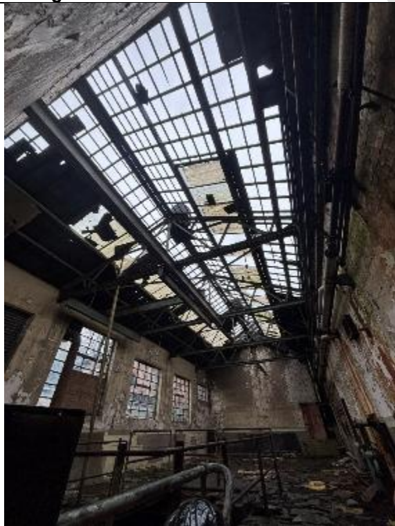
Photograph 15: View of exposed roof within the middle area of the site.
