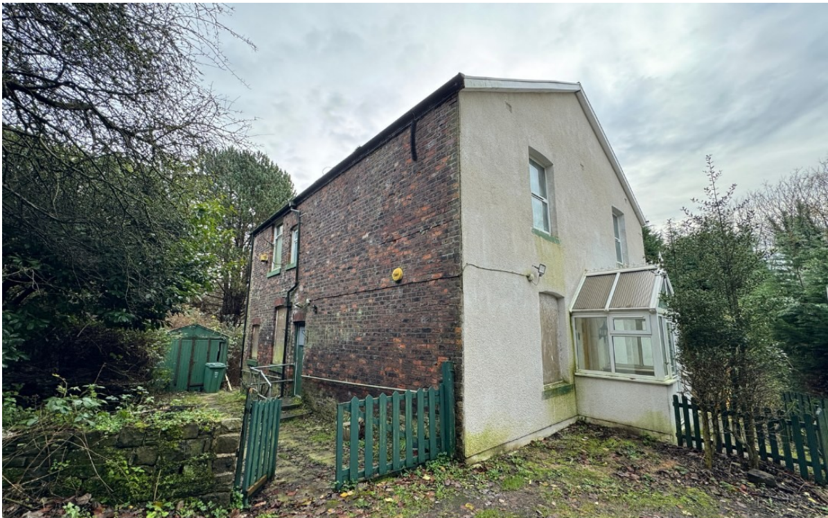
The existing dwelling from Clough Lane: the rendered west gable and brick side elevation
