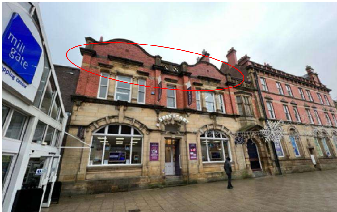
Image 6: Stepped stone projection details above first floor windows to Union Street
