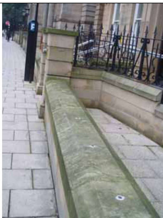
Fig. 51 Railings now missing from Textile Hall
