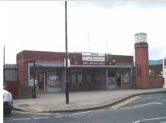
Fig. 23 Bolton Street station
