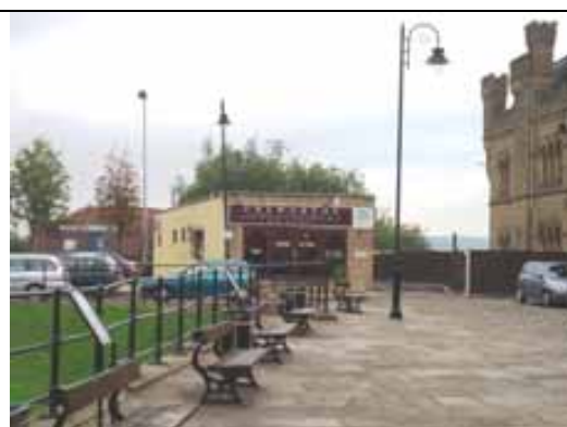
Fig. 122 Single-storey building, Castle Street
