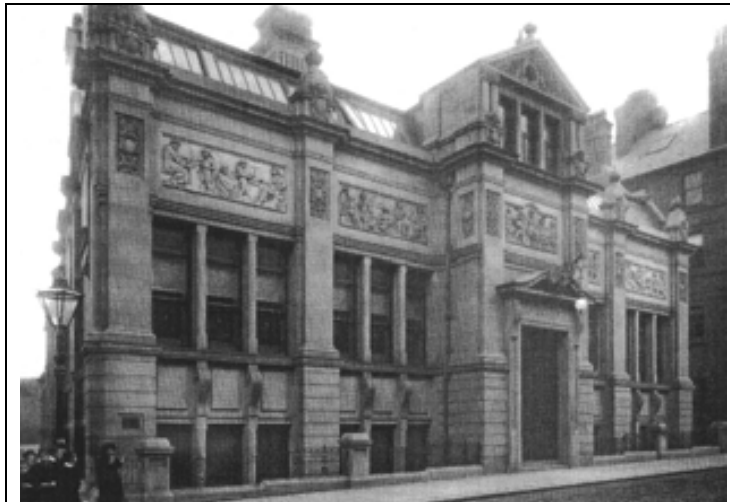
Fig. 44 Technical School, 1805 (Ashworth, 2002)
