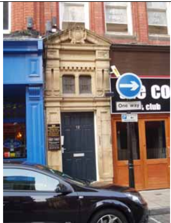
Fig. 55 Door case, Silver Street Chambers (1893)
