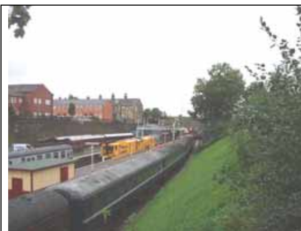
Fig. 7 Bolton Street station
