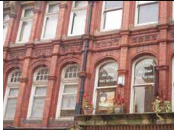
Fig. 58 Brickwork detail, 14-16 Silver Street
