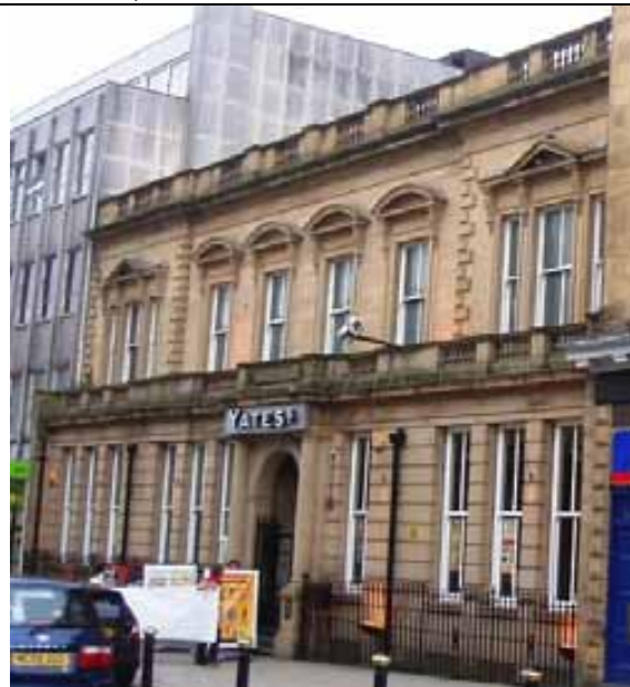
Fig. 102 Historic sashes, 20 Market Street
