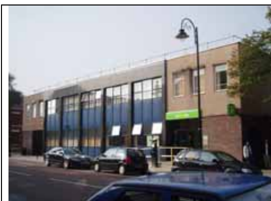
Fig. 121 Job Centre, Silver Street
