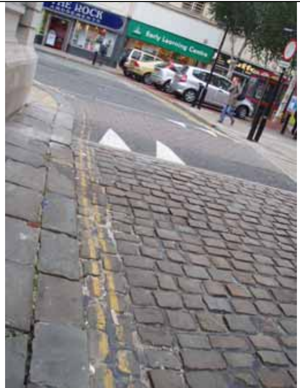
Fig. 72 Setts to north end of Gutter End
