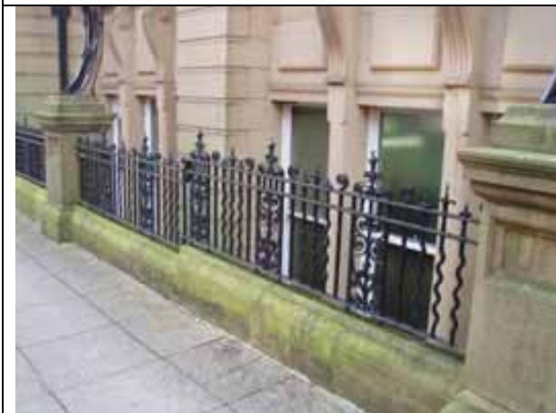
Fig. 82 Railings, School of Arts & Crafts
