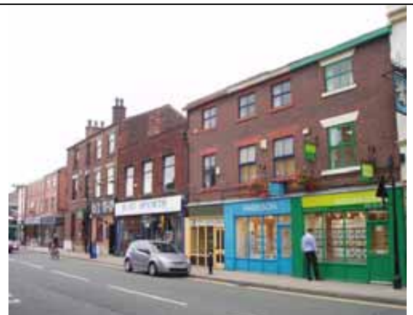
Fig. 70 Reproduction shop fronts at 8-24 Bolton Street
