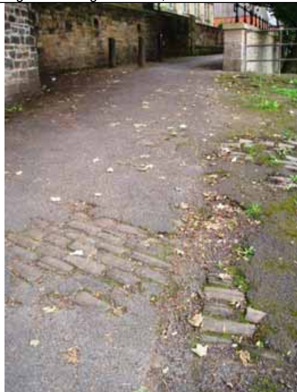
Fig. 73 Setts visible under tarmac, School Brow
