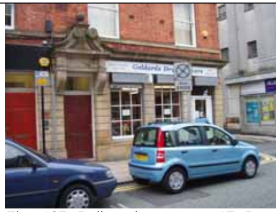
Fig. 107 Roller shutters on 17 Broad Street
