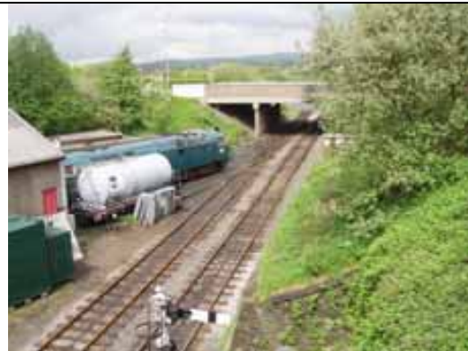
Fig. 24 Railway line immediately west of Castle Street
