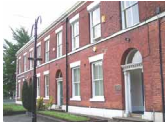
Fig. 60 Sash windows in (L-R) 14-10 Manchester Road
