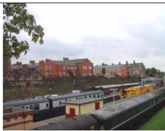
Fig. 8 Bolton Street station
