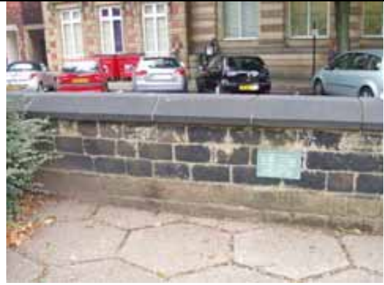
Fig. 59 Churchyard walls, Memorial Gardens, Silver Street
