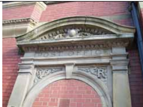
Fig. 56 Stone detail, former GPO, Crompton Street
