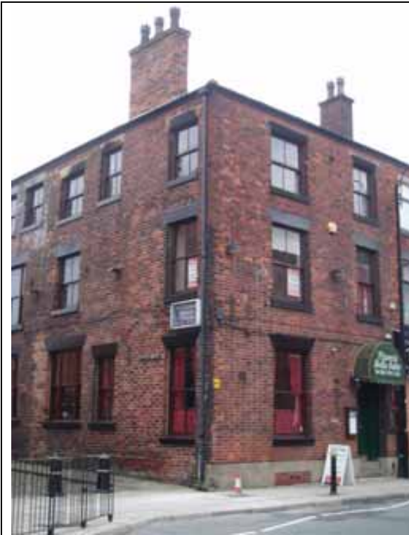
Fig. 119 To let: upper floors of 16 Bolton Street
