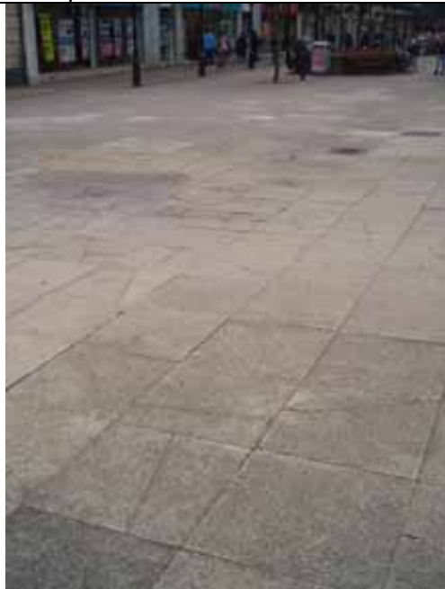
Fig. 77 Paving, Kay Gardens
