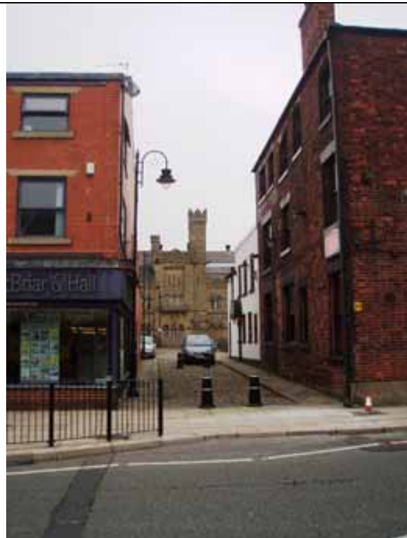
Fig. 91 View from Bolton Street towards the Armoury
