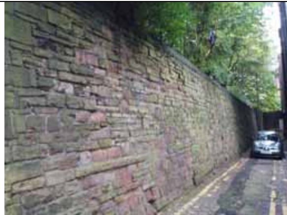
Fig. 16 Rectory wall, rear of 1 The Rock
