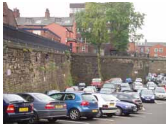
Fig. 25 Bolton Street station walls
