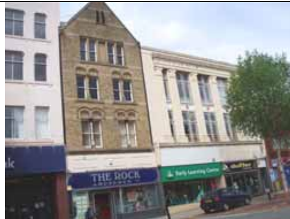
Fig. 109 Modern shop fronts, 13-21 The Rock
