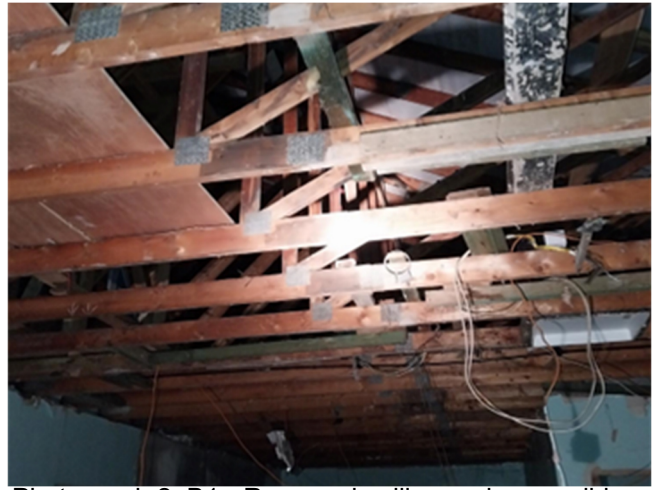
Photograph 2: B1 - Removed ceiling and accessible loft cavity.
