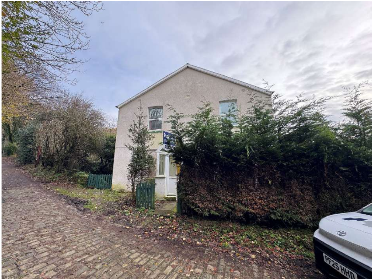
View of property entrance, facing East
