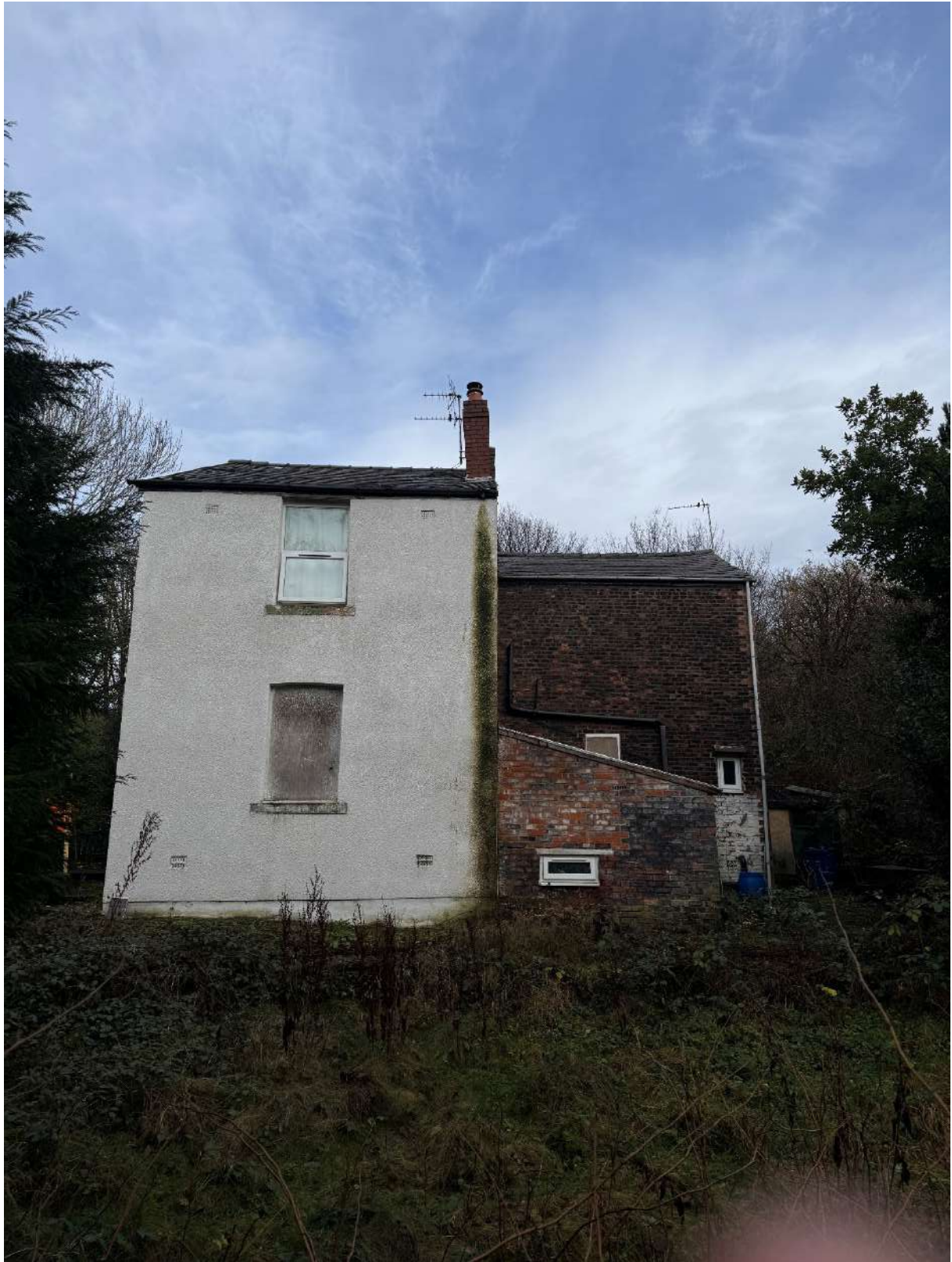
Side view of property, facing South
