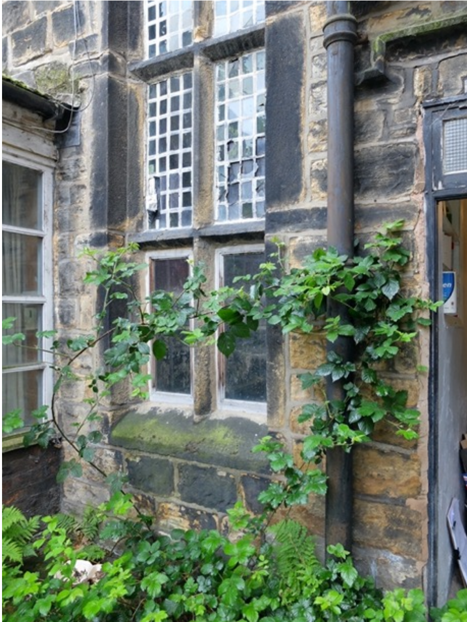
Photo, strap pointing and low level vegetation
