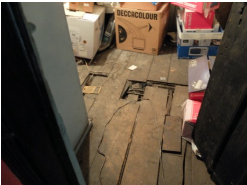
Photo, lifted floorboards
