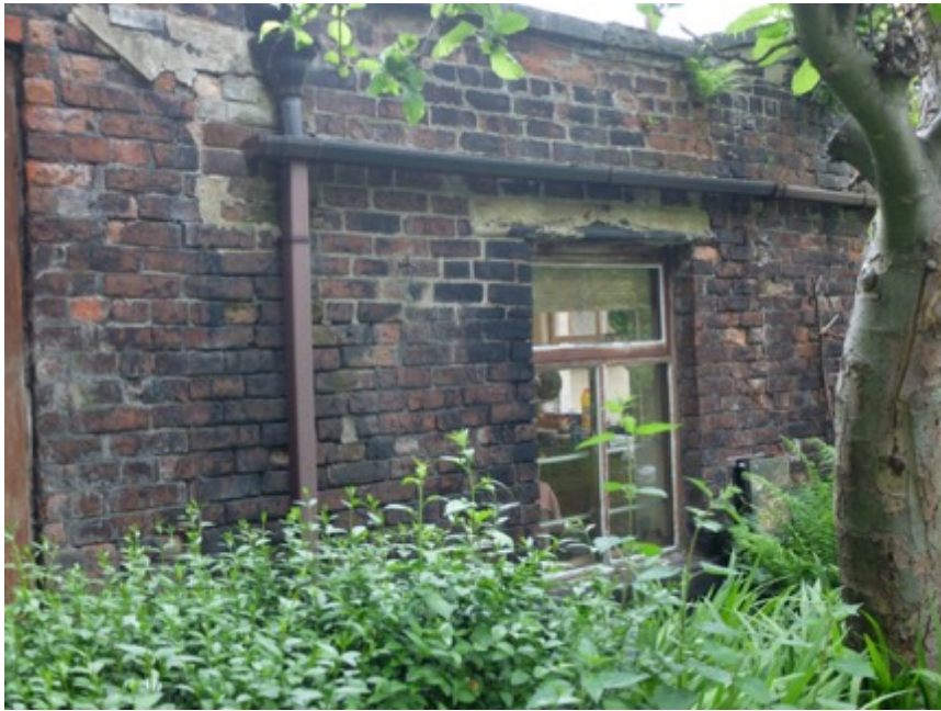
Photo, window with salvaged stone lintel
