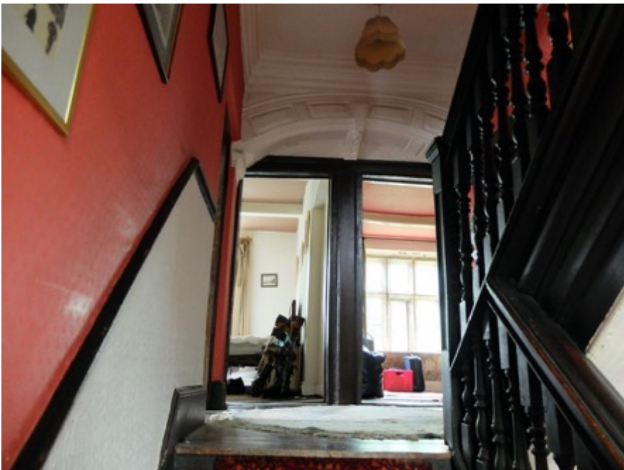
Photo, decorative plaster arch
