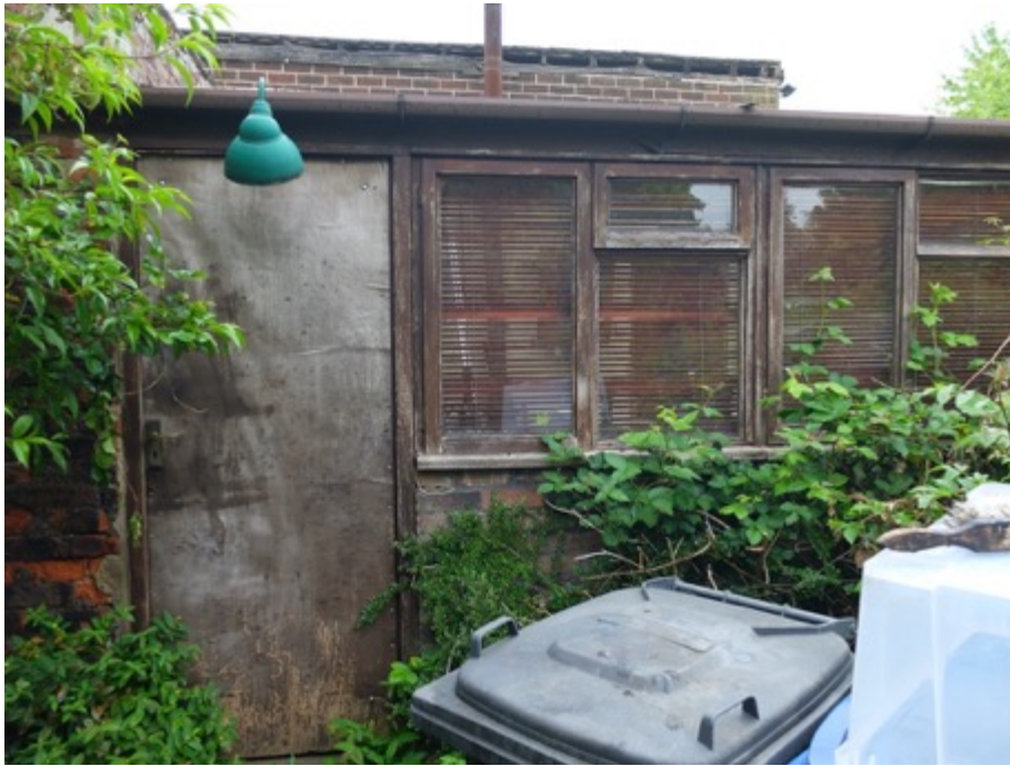
Photo, front wall of workshop
