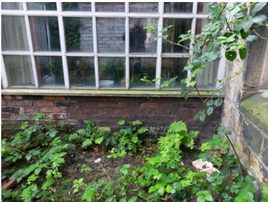
Photo, old and new brickwork
