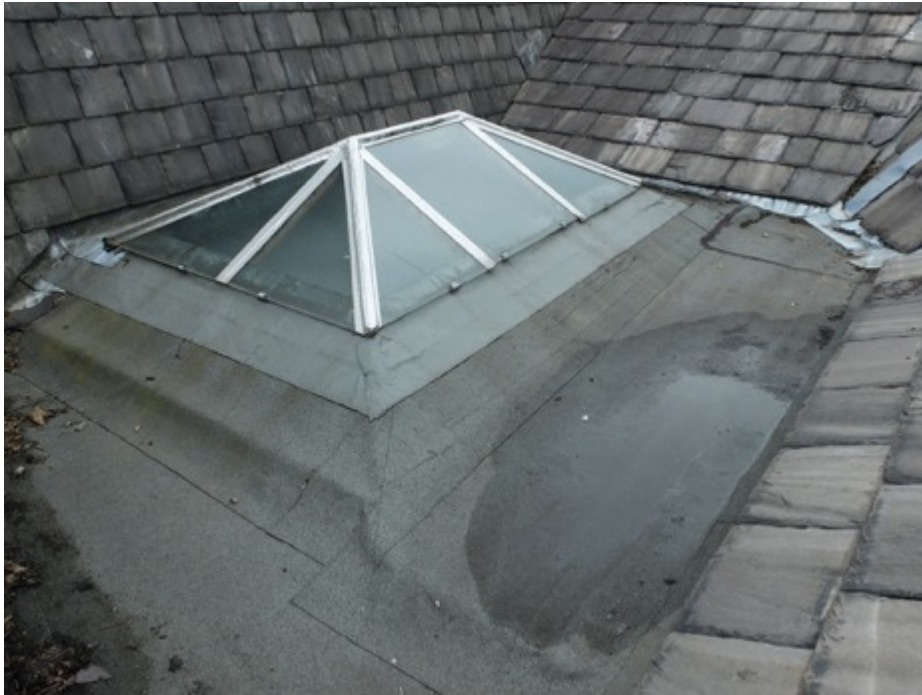
Photo, flat roof to adjoining buildings discharges into gutter on rear elevation
