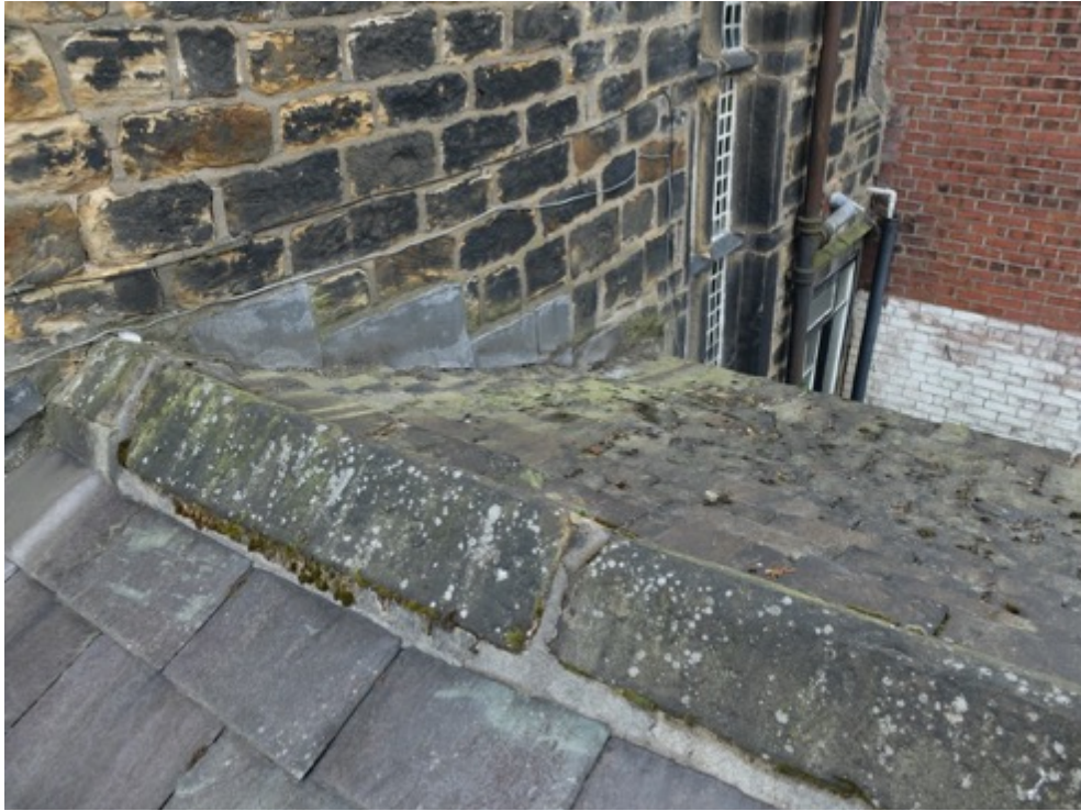
Photo, stone roof over dining room
