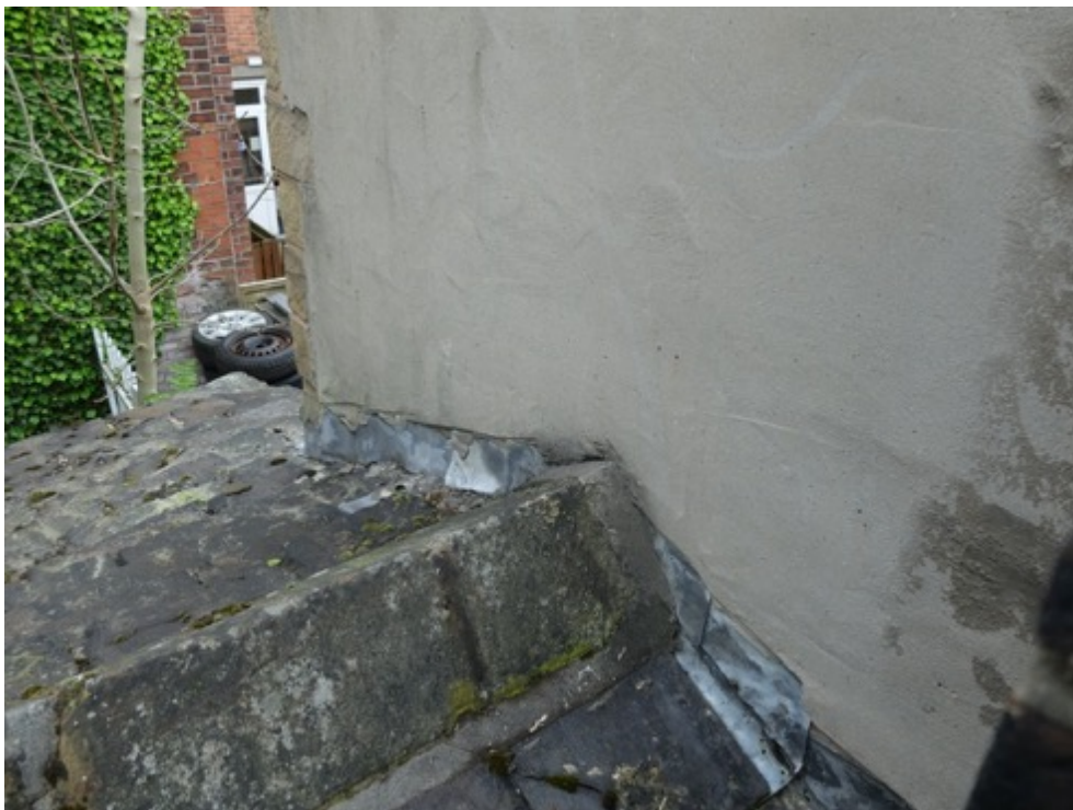
Photo, poor abutment detail with rendered cottage building
