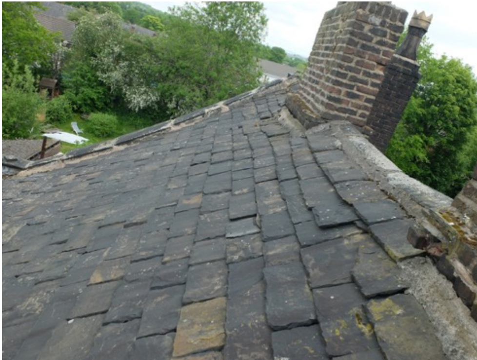
Photo, rear slope
