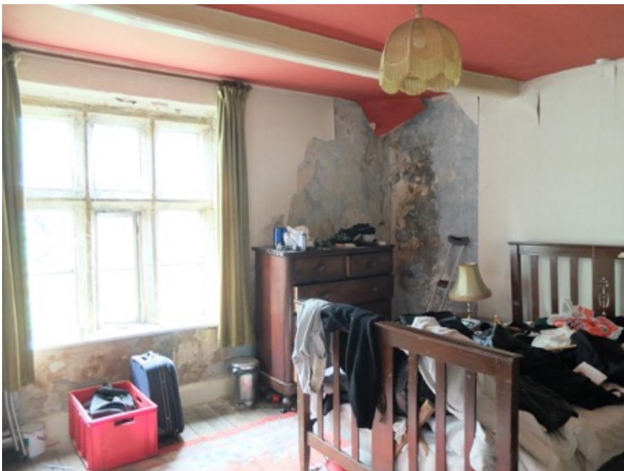
Photo, front left bedroom, ingress to front left corner
