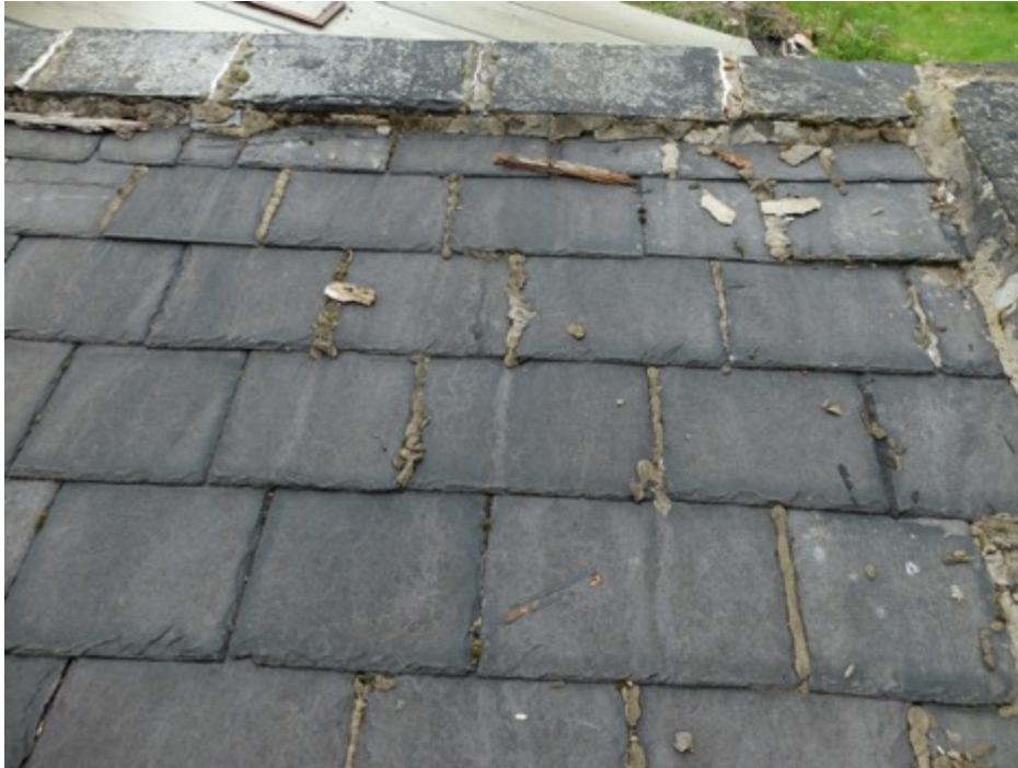
Photo, east slope of roof
