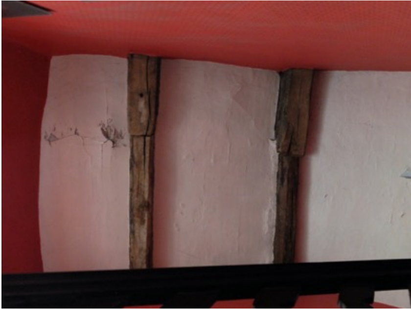
Photo, ceiling over stairs
