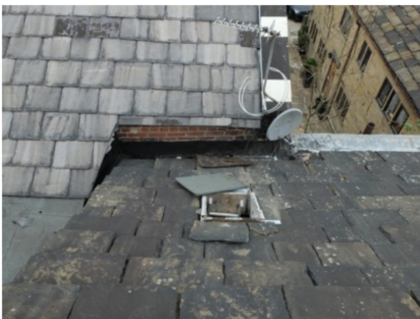
Photo, abutment with rear building
