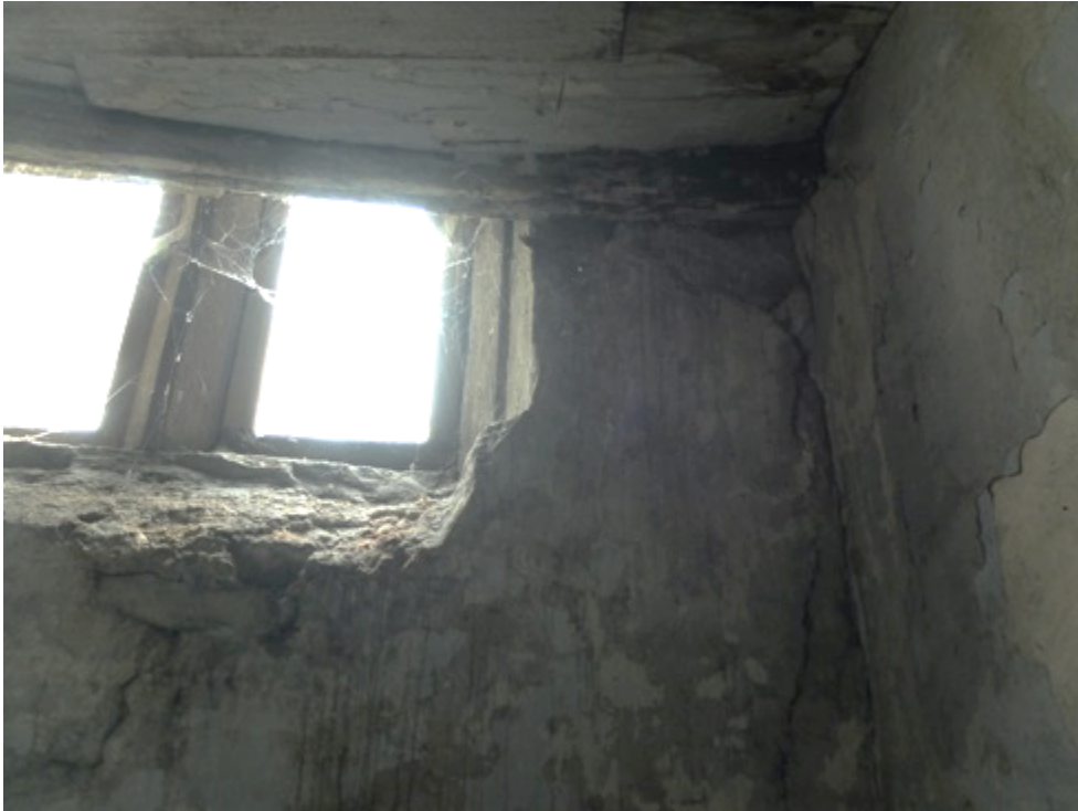
Photo, half landing investigation and repair
