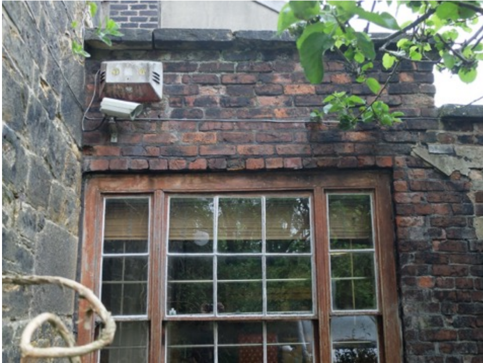
Photo, Large window over kitchen
