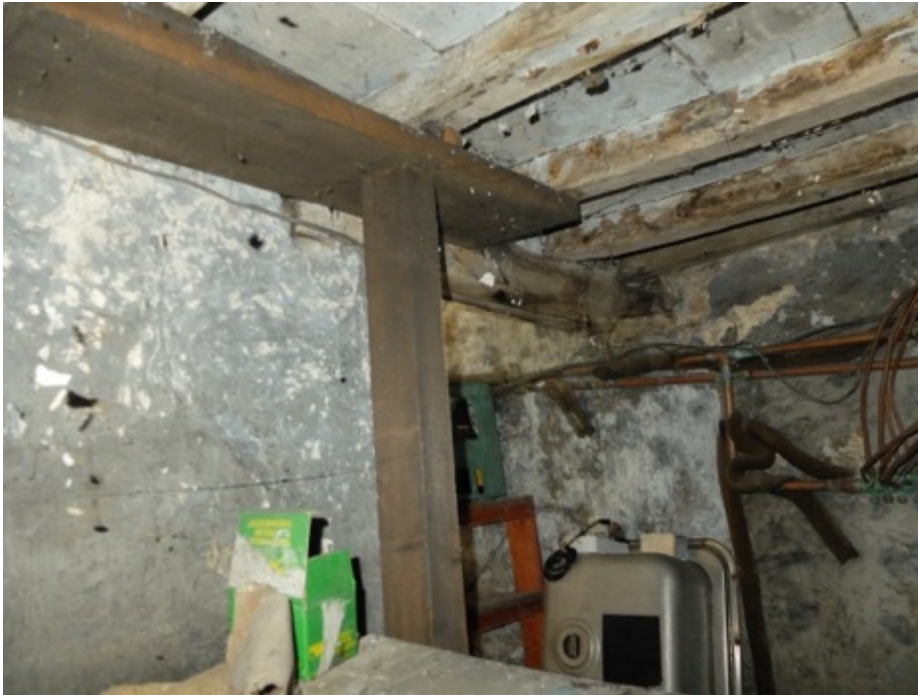
Photo, timber props supporting floors
