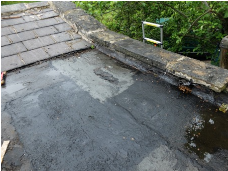
Photo, flat roof and upstands
