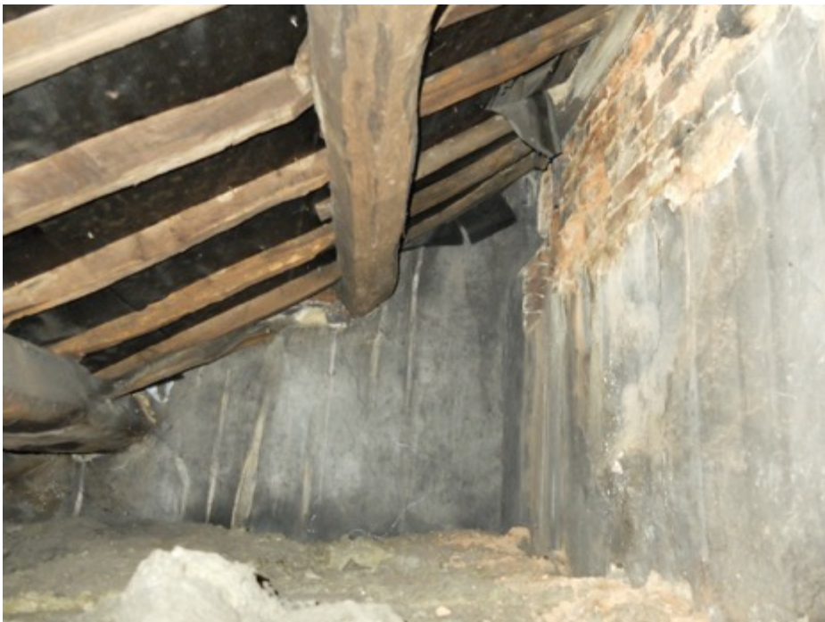
Photo, plastered walls in roof space
