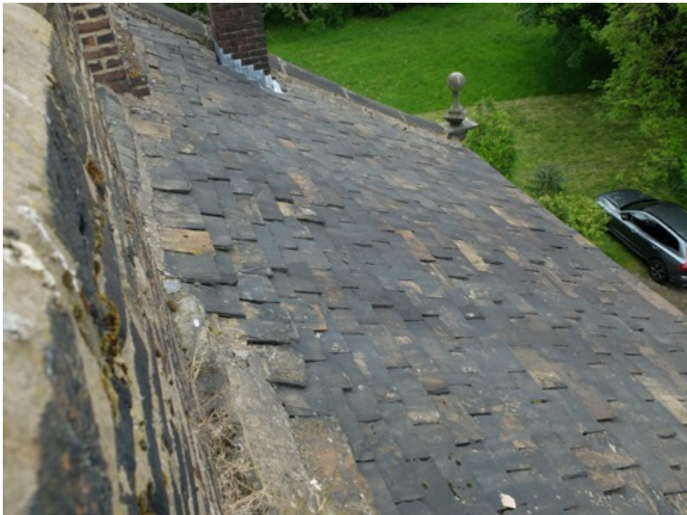
Photo, front slope
