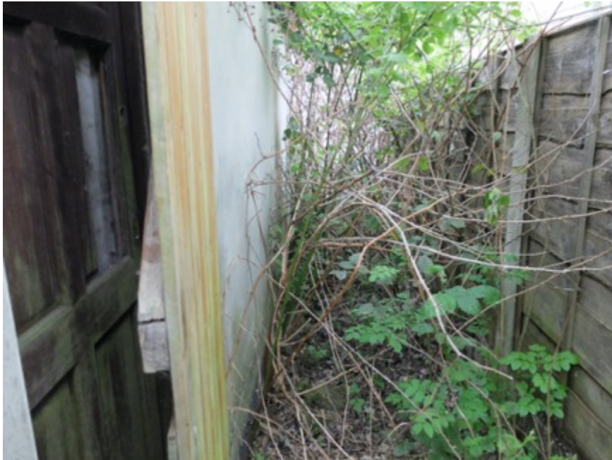
Photo, blocked rear elevation
