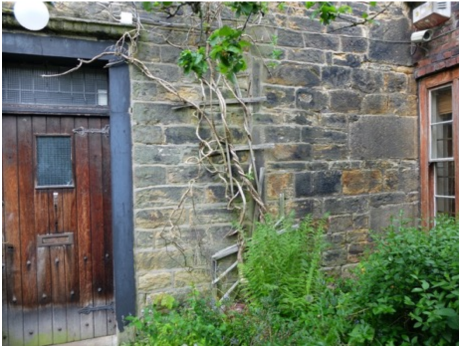
Photo, original door opening
