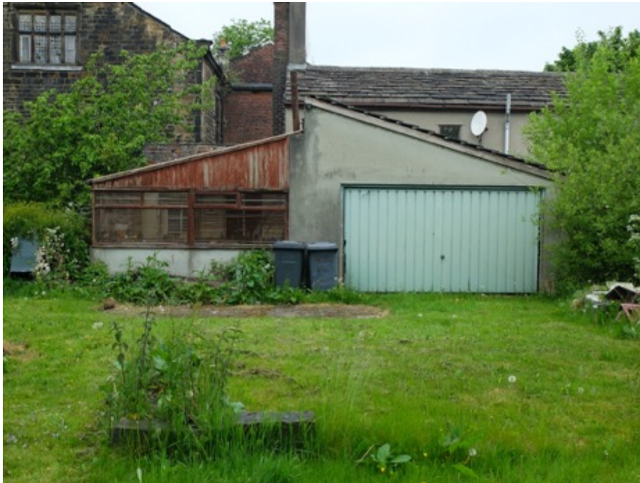
Photo, east elevation
