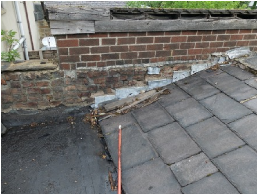
Photo, abutment with wall
