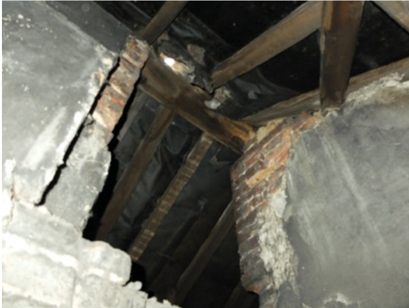
Photo, view of roof space
