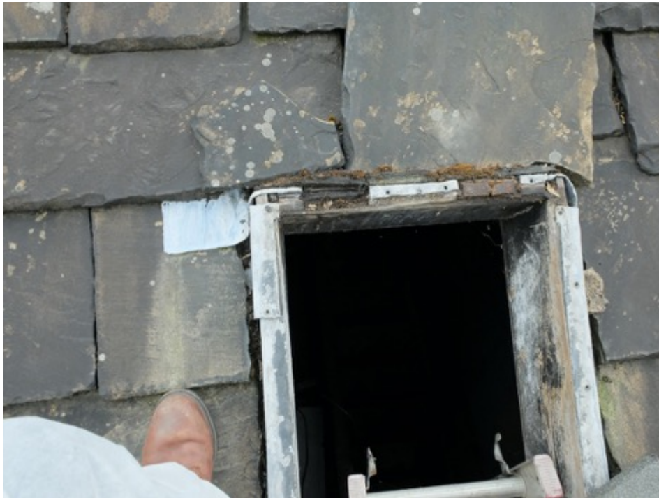
Photo, Access trap on to roof
