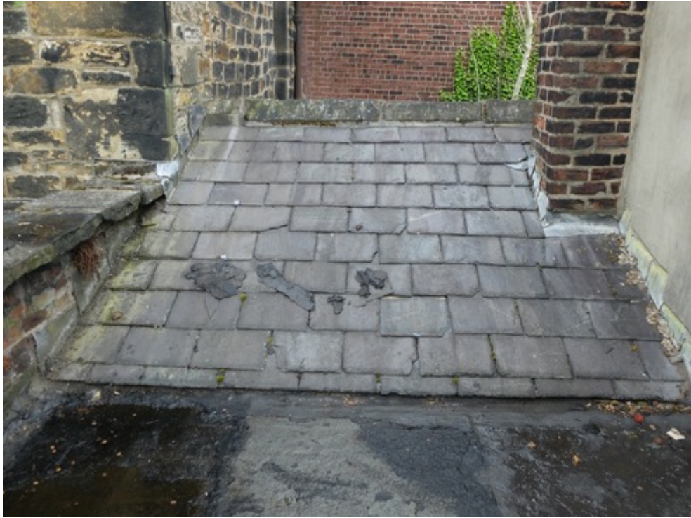
Photo, west slope of slated roof
