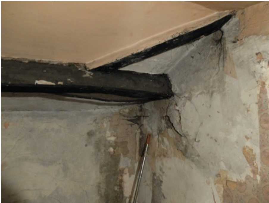
Photo, roof and rear wall abutment
