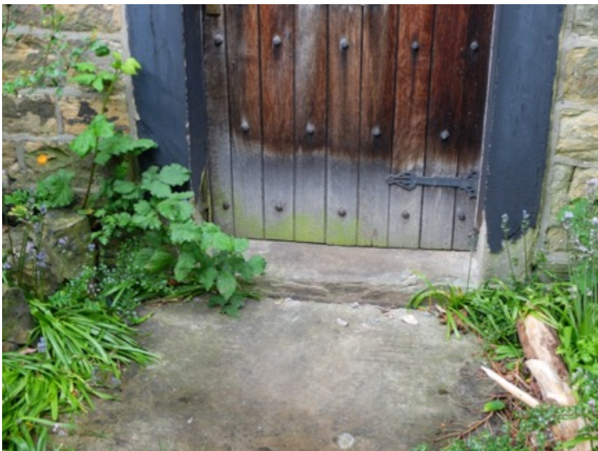
Photo, Erosion of stone and lichen moss to main door
