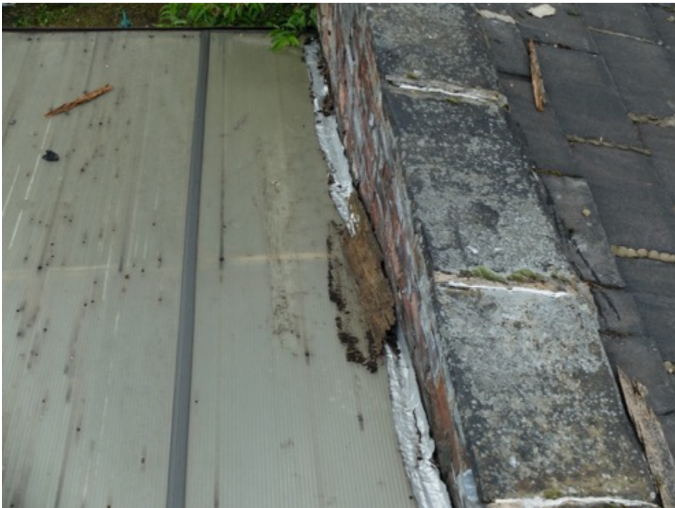
Photo, workshop roof
