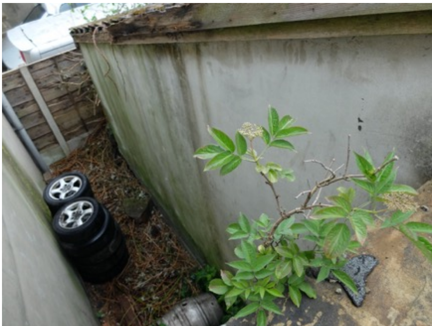
Photo, no access west elevation
