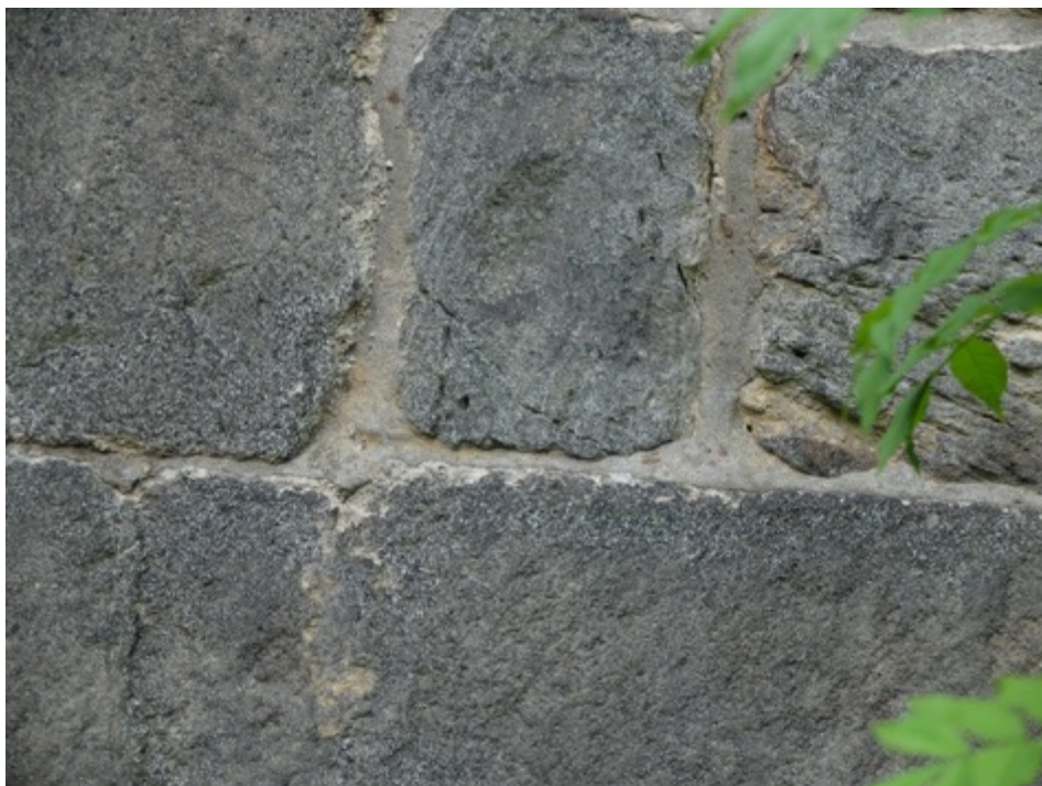
Photo, examples of sand and cement pointing
