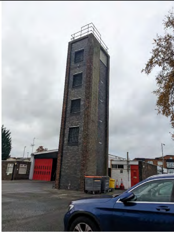
Figure 7 – View south west from the north eastern site section showing the main fire station building and training tower
