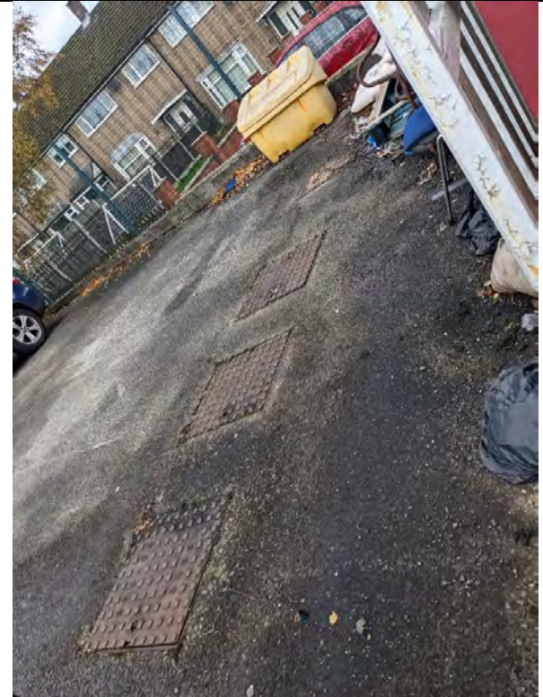
Figure 4 – Looking north west from the north easter site section showing suspected interceptors
