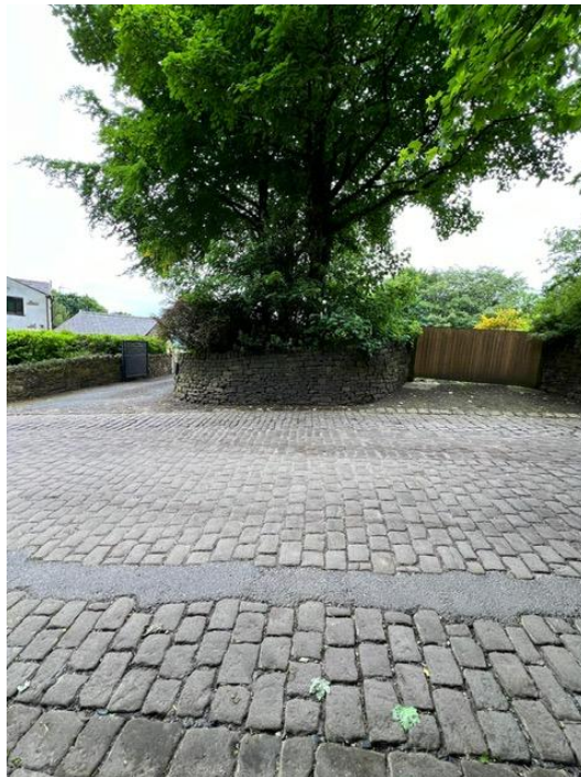
View to the main gates to Ivy Bank
