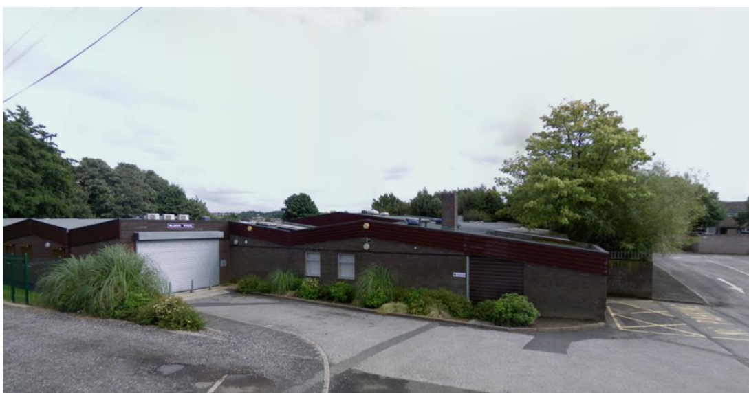
Figure 13- Millwood School, 2008, with the footpath seen as the tarmac path to the right of the buildings
