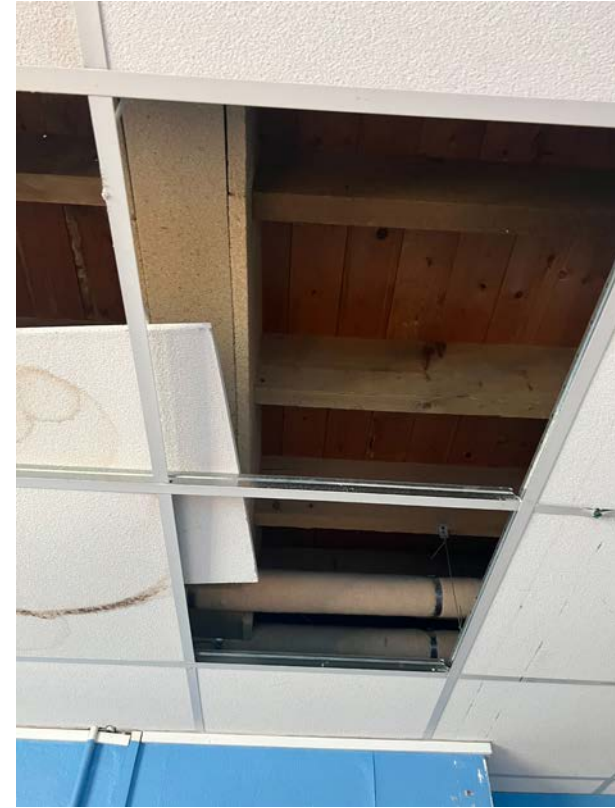
PLATE 8: Ground floor mezzanine ceiling construction.
