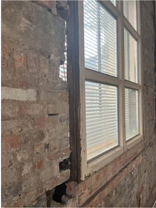
PLATE 5: Secondary glazing panels within the main banking hall, south wall.
