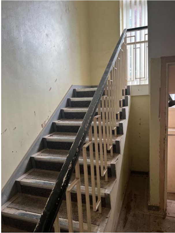
PLATE 9: Later stair to north internal wall.
