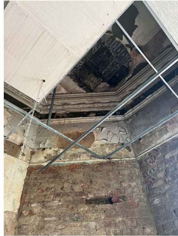
PLATE 16: Retained ceiling plasterwork and cornice at first floor.
