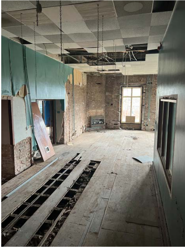
PLATE 13: First floor main space to south side of building looking east.
