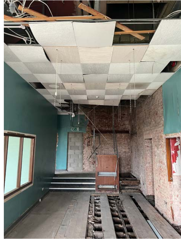
PLATE 14: First floor main space to south side of building looking west
