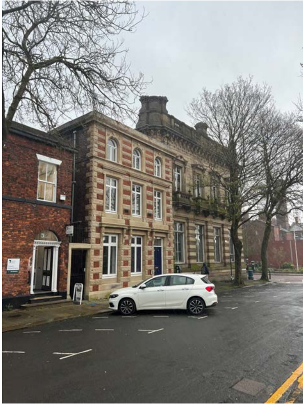
PLATE 3: View north-east from Bank Street showing the former annex, Bank Chambers, building.
