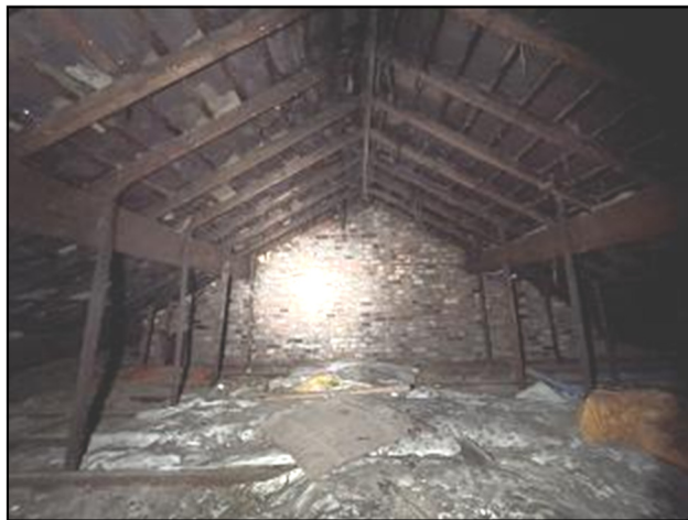
Plate 1 Main roof void
