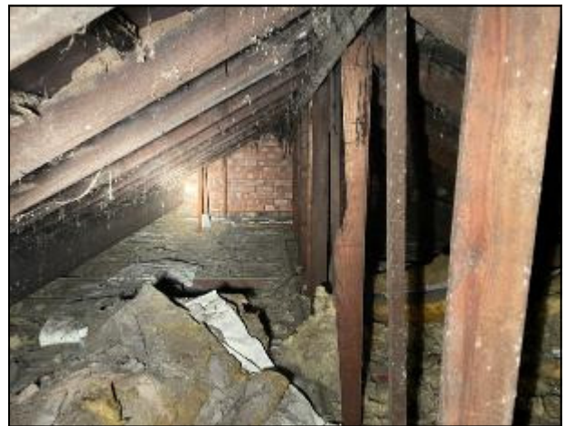
Plate 2 Outtrigger roof void
