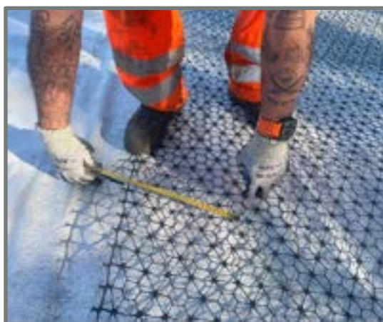
Geogrid and term install, 300mm overlay
