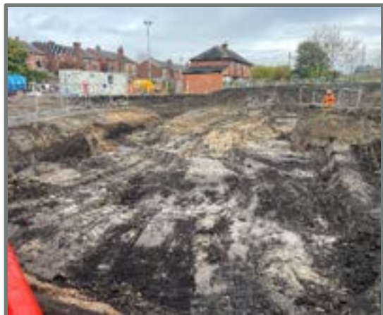
Base of excavation
