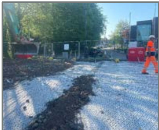
Geogrid and stone install
