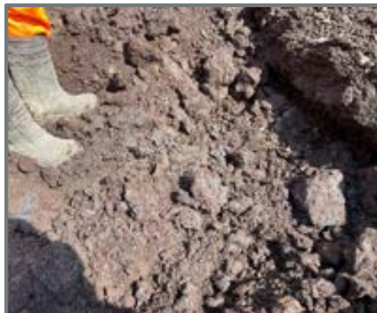
Soft material removed
