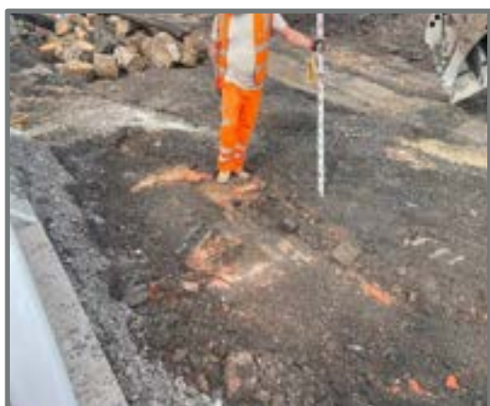
Check layer install using lazer level
