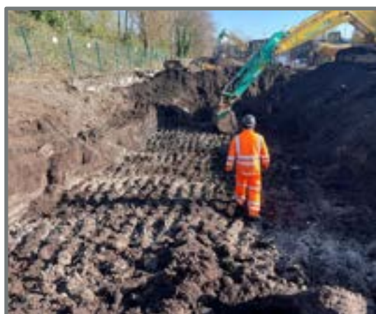
Base of excavation
