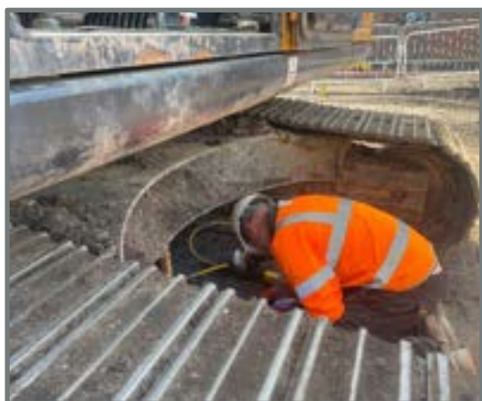
Plate load test
