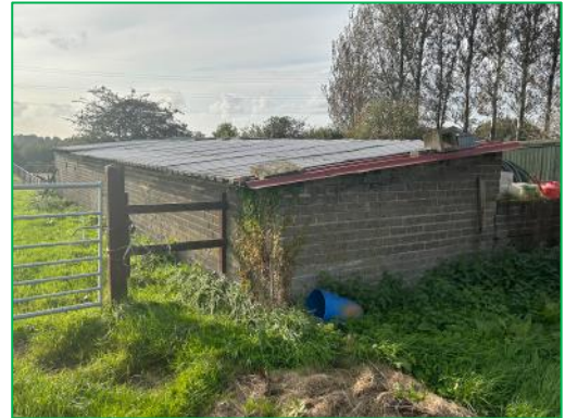
The south and east elevation of the chicken coop
