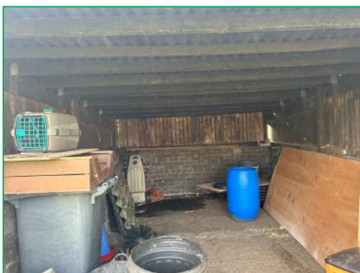
The internal space in the shed
