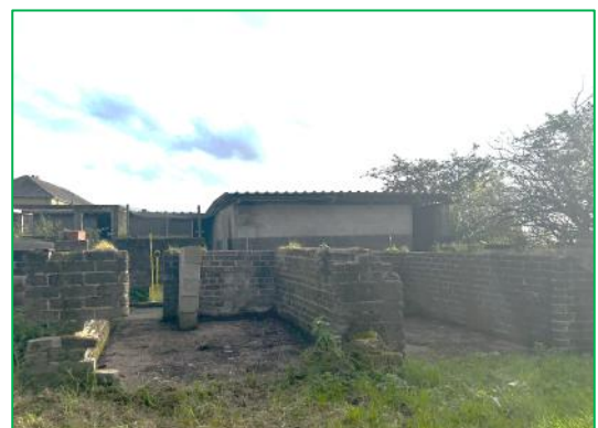
The demolished, western side of the shed
