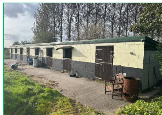
The south elevation of the stables
